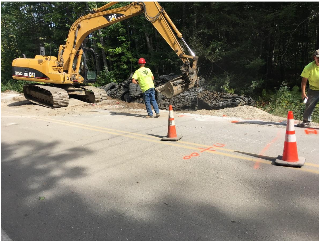
Last blast of the day for water main extension at STA 17+25 just north of stream culvert.
