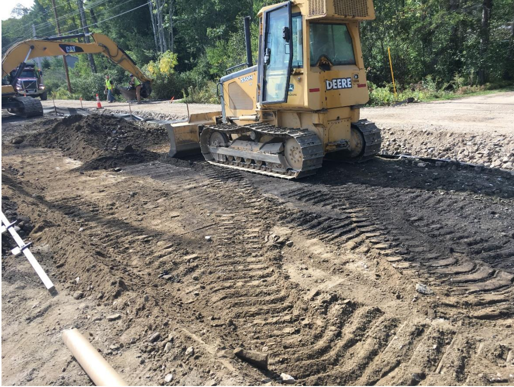
Firm granular subgrade near STA 42+50 (across from driveway for 80 Middle Road).
