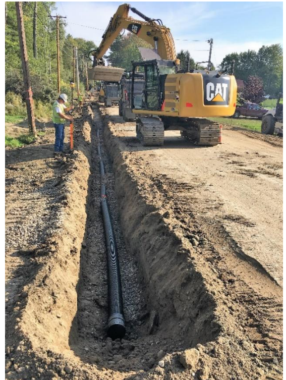
North outlet of underdrain installation on left at STA 41+88 and southern upland terminus of underdrain at STA 39+70. Total length is 220 feet.
