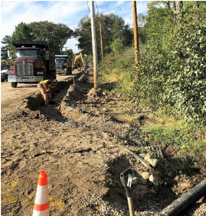
North outlet of underdrain installation on left at STA 41+88 and southern upland terminus of underdrain at STA 39+70. Total length is 220 feet.
