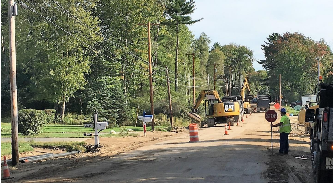
Using 2 excavators to place crushed stone bedding around pipe followed by gravel backfill.
