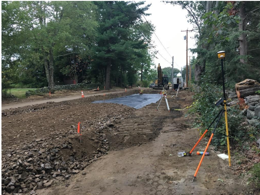
Photograph 8 - Tuesday, September 19 th – Finishing up box cut in west lane at STA 46+00 and placing Type D gravel to match up with east lane near the end of the day.
