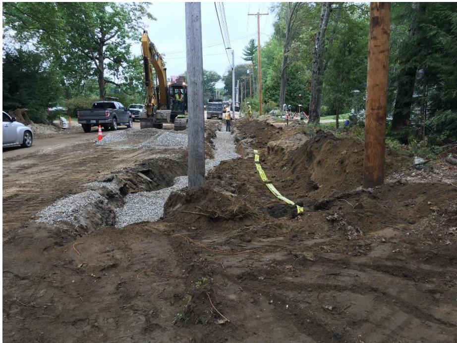
Photograph 6 - Monday, September 18 th - Installing 6-inch underdrain and 4-inch gas main in adjacent trenches south of STA 47+30. Pole 316 in foreground.
