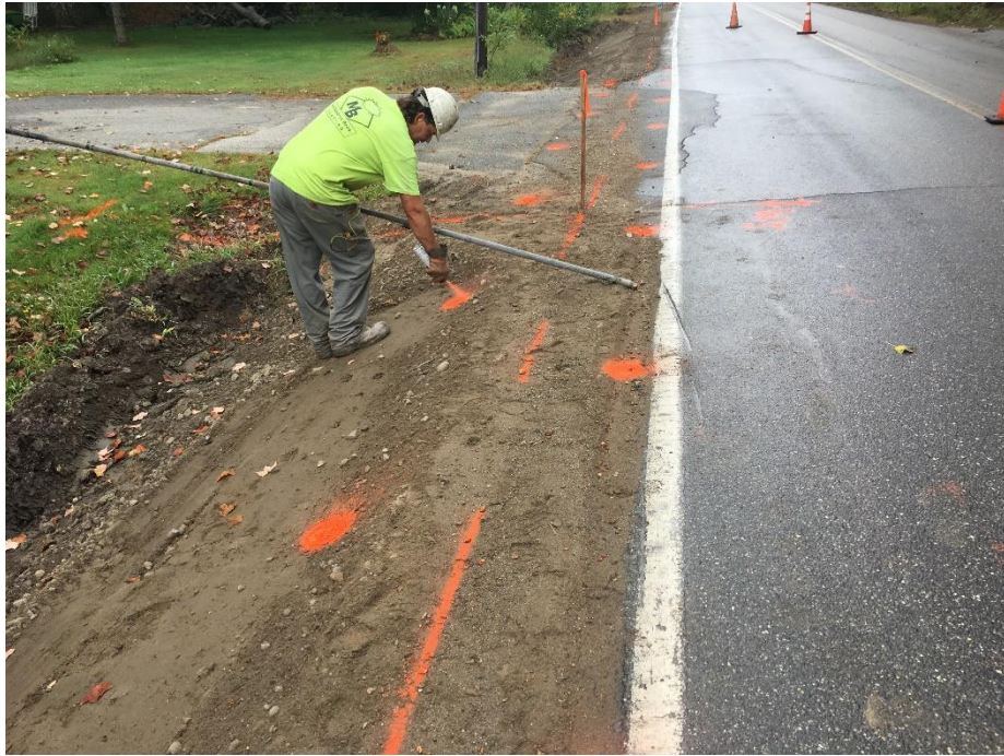
Photograph 5 – Monday, September 18 th – McGoldrick laying out drilling locations prior to blasting for water main extension south of Shirley Lane.
