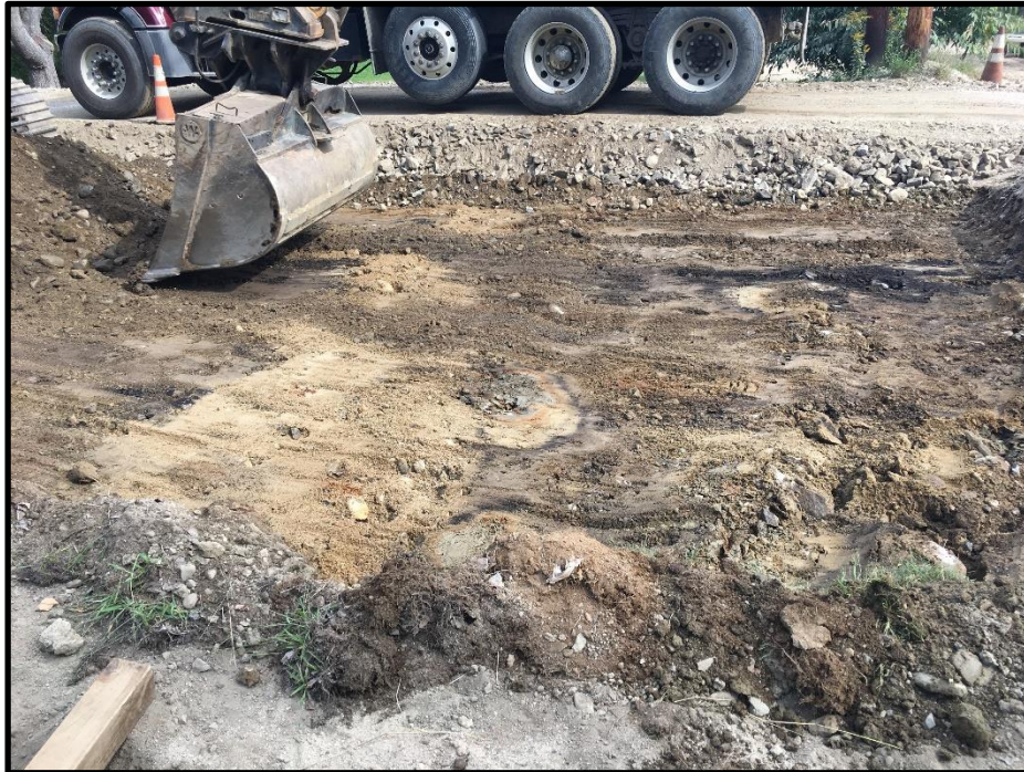
Photograph 1 – Thursday, September 14 th - Exposed subgrade near STA 28+50, Left in the segment from STA 27+00 to STA 31+00 originally proposed for partial box cut. Excavated subgrade shown is near the interface of existing gravel and original subgrade consisting mostly of a silty sand with clay lenses.
