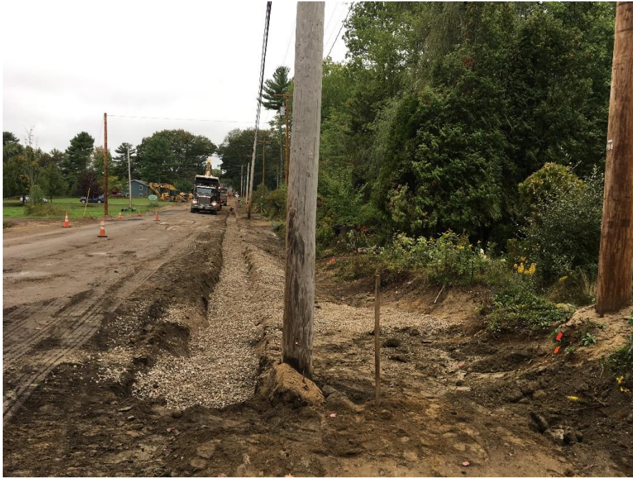
Photograph 9 – Wednesday, September 20 th – Installed 6-inch underdrain from STA 44+30 to STA 41+88. Pole #314 in foreground
