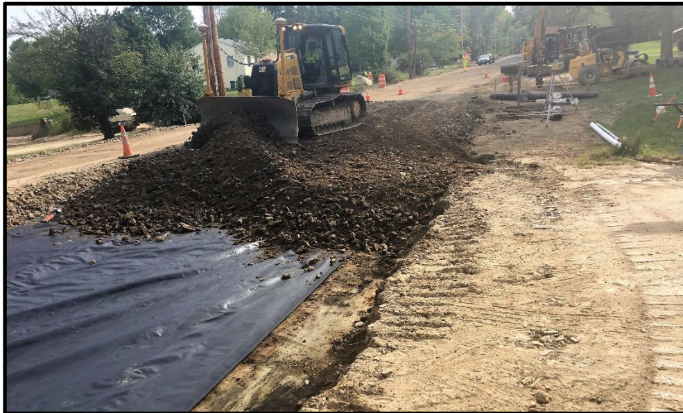
Photograph 2: Thursday, September 14 th - New Type D gravel being placed on geotextile fabric in front of Range Way at STA 28+00, Left. Gravel of exceptional quality (well graded with good angularity).
