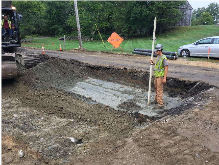
Photograph 7 – Tuesday, September 19 th - After peeling away pavement, Storey Brothers starting to box cut road in east lane at STA 49+20 (in front of 95 Middle Road) working southward from east to west.
