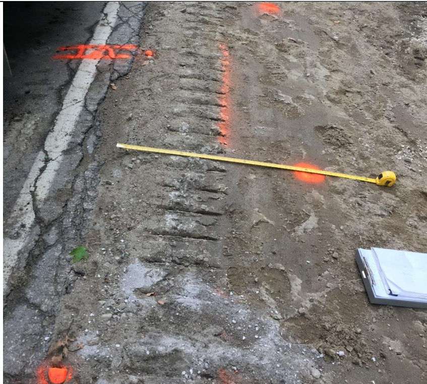
Photograph 10 – Wednesday, September 20 th – Layout of alternating drill locations 3 feet wide and 7 feet longitudinally at Waterfall Way.
