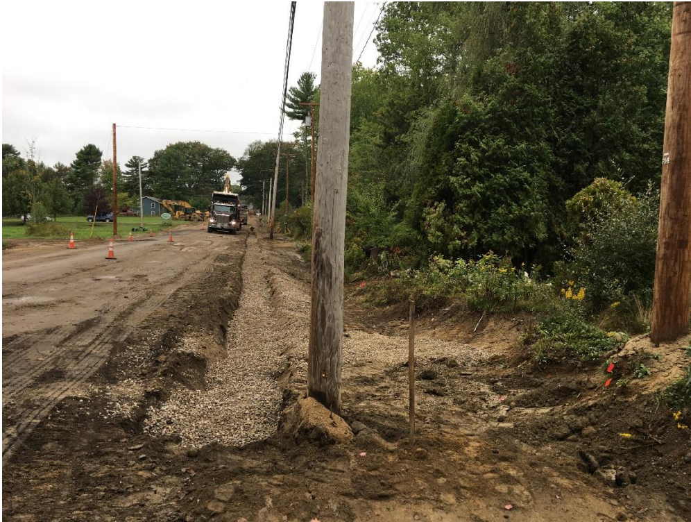
Installed 6-inch underdrain from STA 44+30 to STA 41+88. Pole #314 in foreground.
