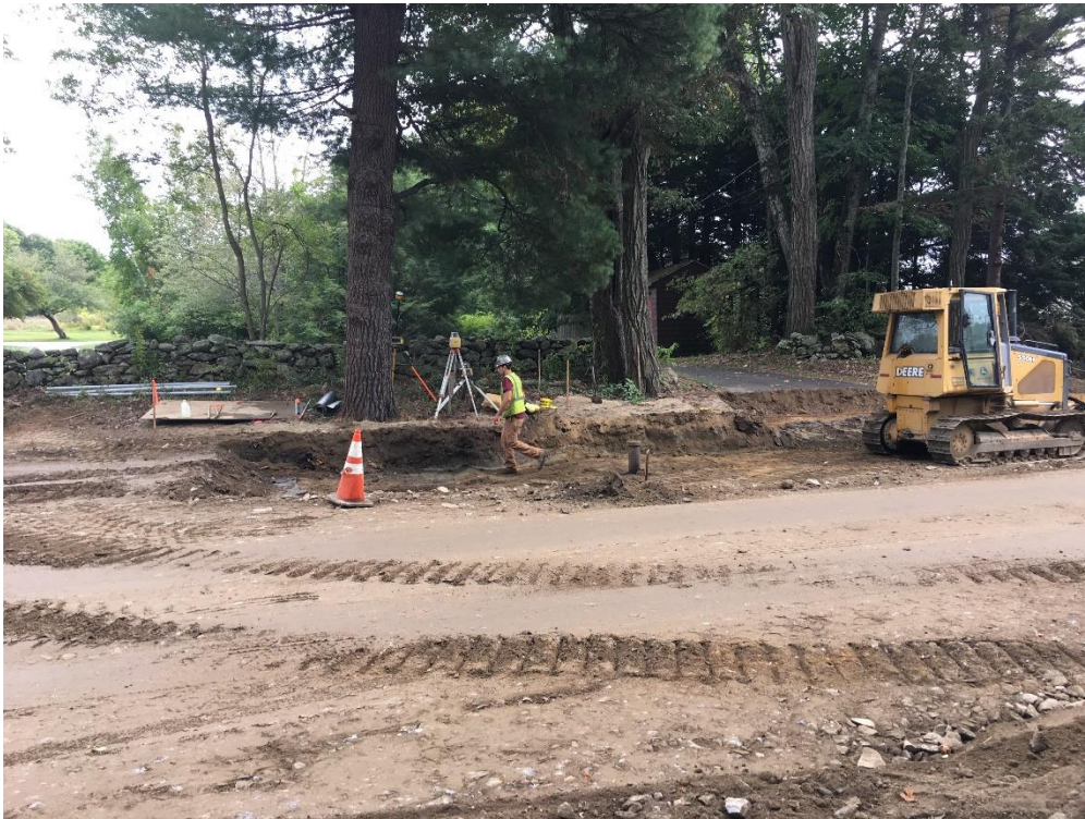
Starting eastern half of box cut at STA 46+00 (completed western half in foreground). Dozer used to grade and "proof roll" the subgrade prior to placement of geotextile fabric.
