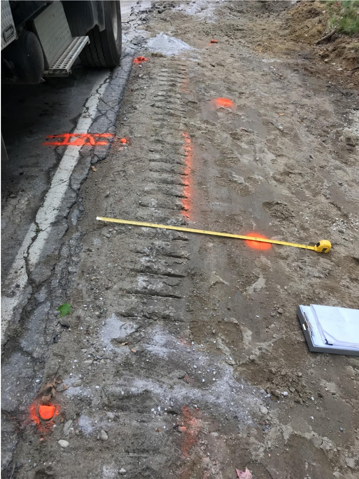
Layout of alternating drill locations 3 feet wide and 7 feet longitudinally at Waterfall Way.
