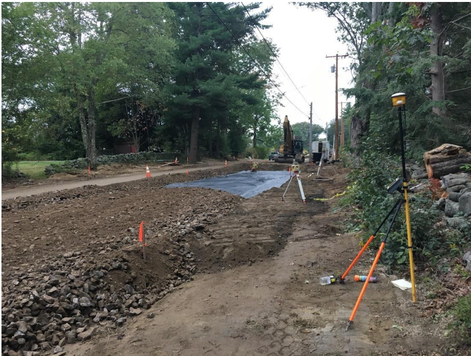
Finishing up box cut in west lane at STA 46+00 and placing Type D gravel to match up with east lane near the end of the day.
