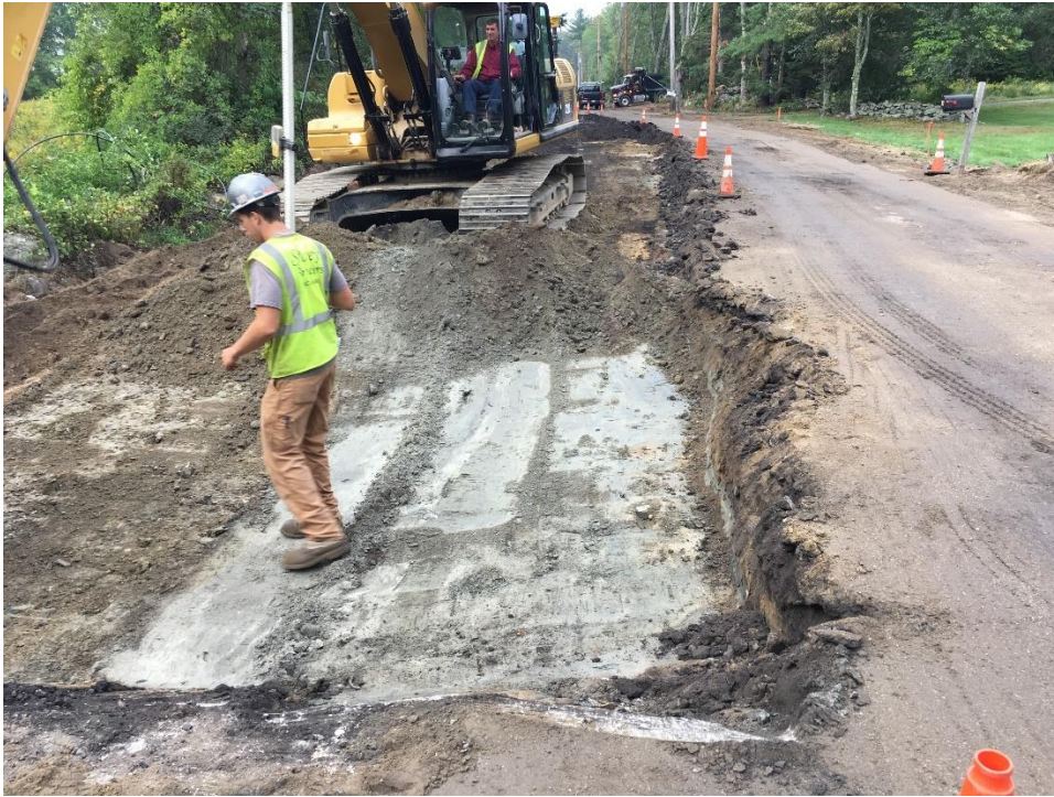
After peeling away pavement, Storey Brothers starting to box cut road in east lane at STA 49+20 (in front of 95 Middle Road) working southward from east to west.
