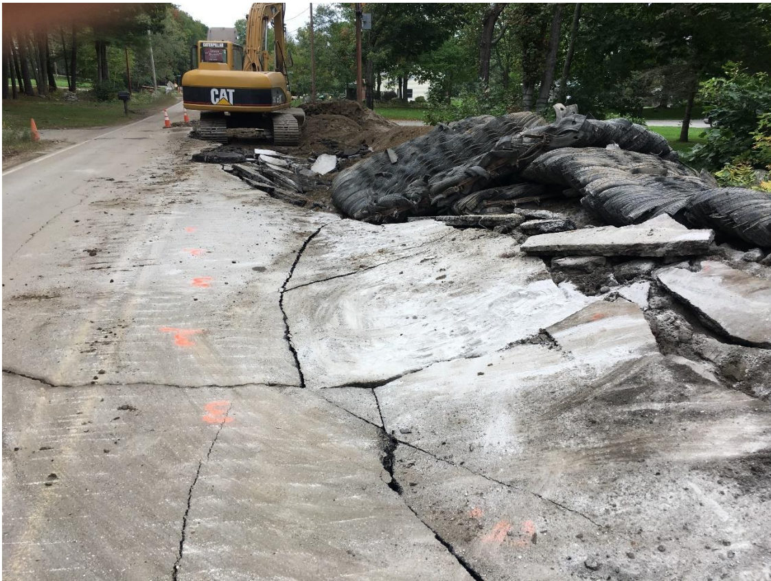
Cleaning up after blast near STA 22+50. Overburden typically 3 feet (see numbers at left).
