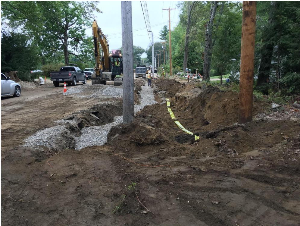
Installing 6-inch underdrain and 4-inch gas main in adjacent trenches south of STA 47+30. Pole 316 in foreground.
