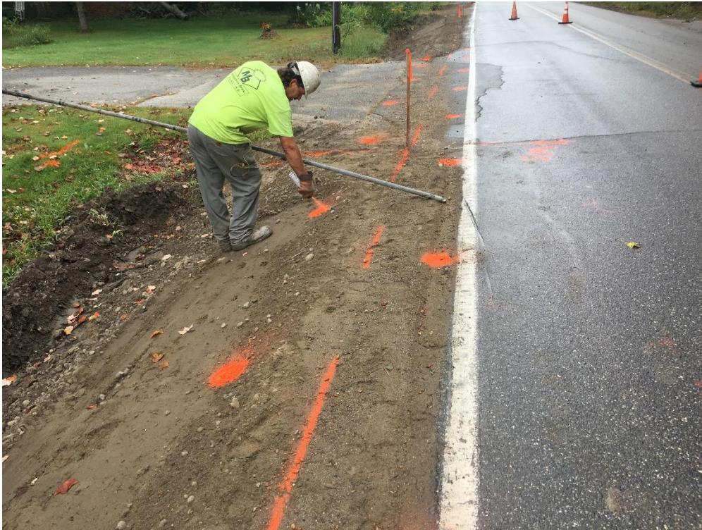
McGoldrick laying out drilling locations prior to blasting for water main extension south of Shirley Lane.
