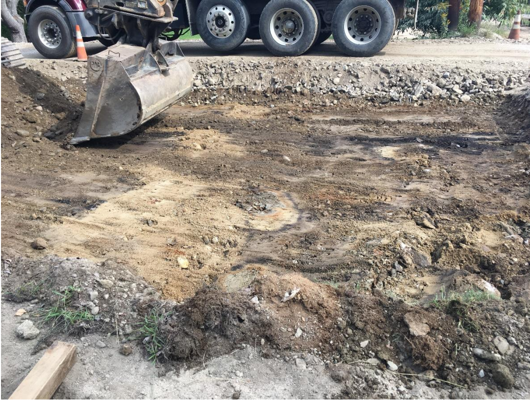
Exposed subgrade near STA 28+50, Left in the segment from STA 27+00 to STA 31+00 originally proposed for partial box cut. Excavated subgrade shown is near the interface of existing gravel and original subgrade consisting mostly of a silty sand with clay lenses.
