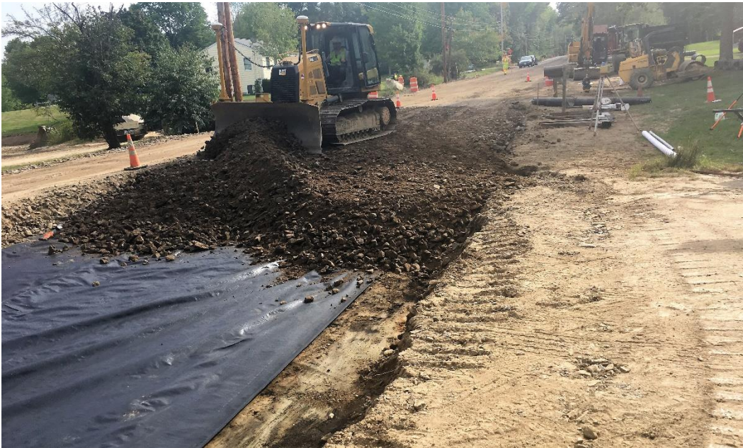
New Type D gravel being placed on geotextile fabric in front of Range Way at STA 28+00, Left. Gravel of exceptional quality (well graded with good angularity).
