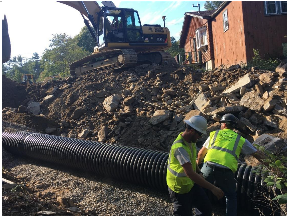
Photograph 10 – Wednesday, September 13 th – Installing the culvert extension downstream of the elbow in the drainage easement behind 55 Middle Road.
