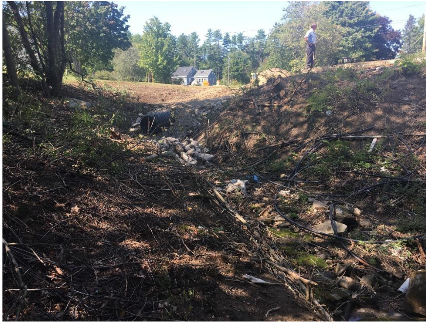
Photograph 5 – Monday, September 11 th – At the drainage easement at 55 Middle Road a 45-degree elbow will be added from this point where the existing drainage way turns so that the culvert can be extended.
