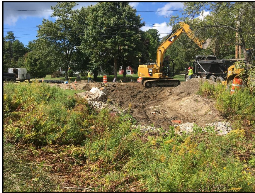
Photograph 4 - Friday, September 8 th – Installing the cross culvert near STA 26+85 and beginning the work on the drainage easement between 53 and 55 Middle Road.
