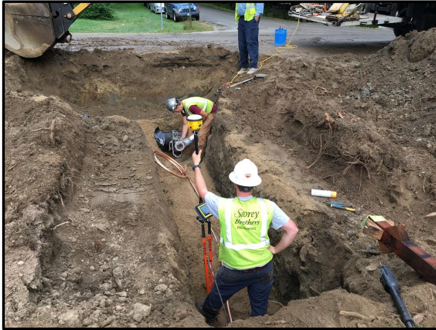
Photograph 1 – Thursday, September 7 th - Tapping installed (but empty) section of water main extension for water service at 55 Middle Road near STA 27+60, RT (across the road from Rangeway).
