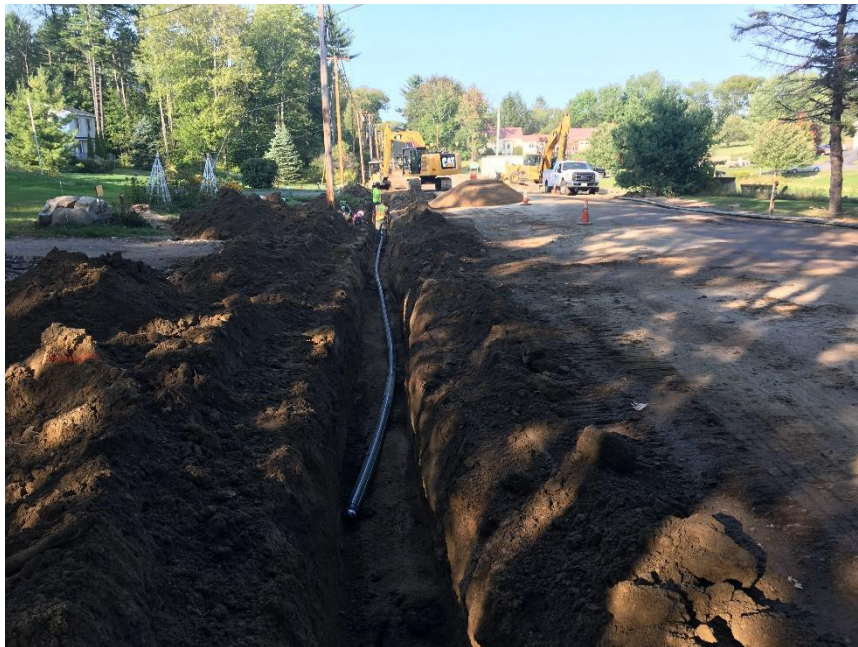
Photograph 6 - Monday, September 11 th - Southern extent of the gas line installation near the end of day at 37+75. Crew had to skip from STA 45+25 to STA 47+25 due to ledge. Ledge to be removed Wednesday.
