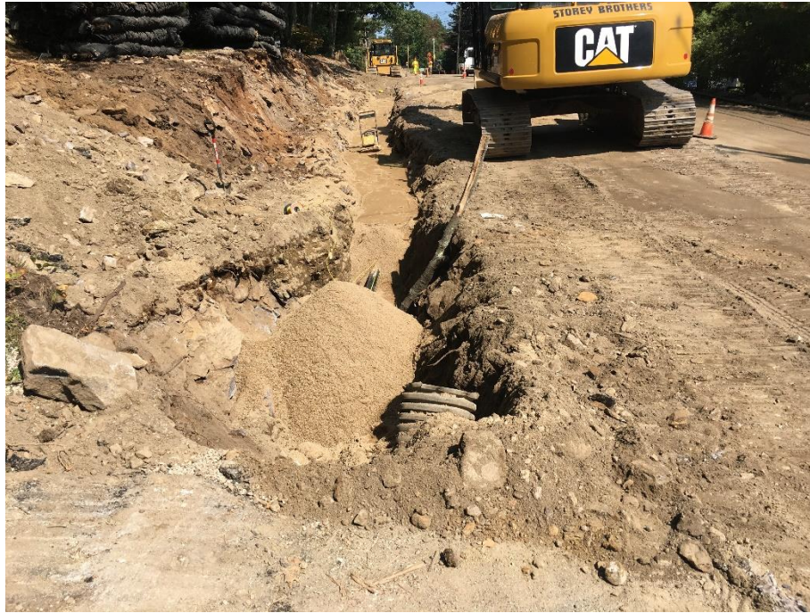
Photograph 7 – Tuesday, September 12 th - Installed section of gas main between 70 and 72 Middle Road previously blasted.
