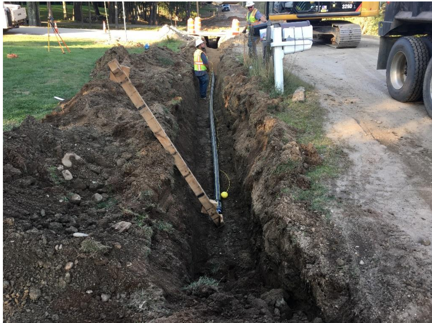
Photograph 8 - Tuesday, September 12 th – Southern extend of gas main installation at STA 27+30 (54 Middle Road) at end of day.
