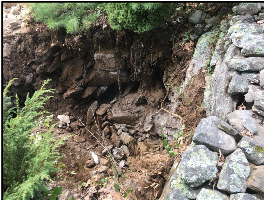
Photograph 2: Thursday, September 7 th - Additional ledge had to be removed with a hoe ram attachment to excavator to install the final water service (at 72 Middle Road) near STA 36+60, LT.
