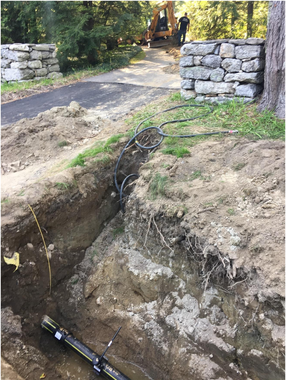
Installing the service connection to the previously installed (uncharged) gas main onto the Knowles property at 148 Middle Road.
