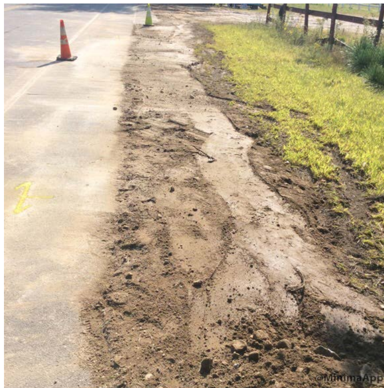
Backfill brought to grade and compacted.
