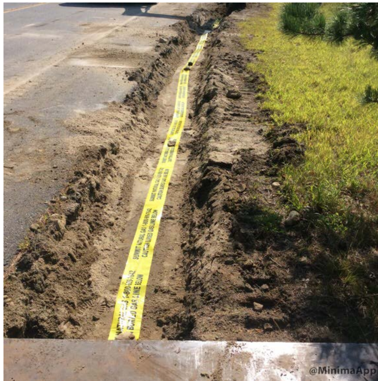
Compacted backfill with warning tape in trench area.
