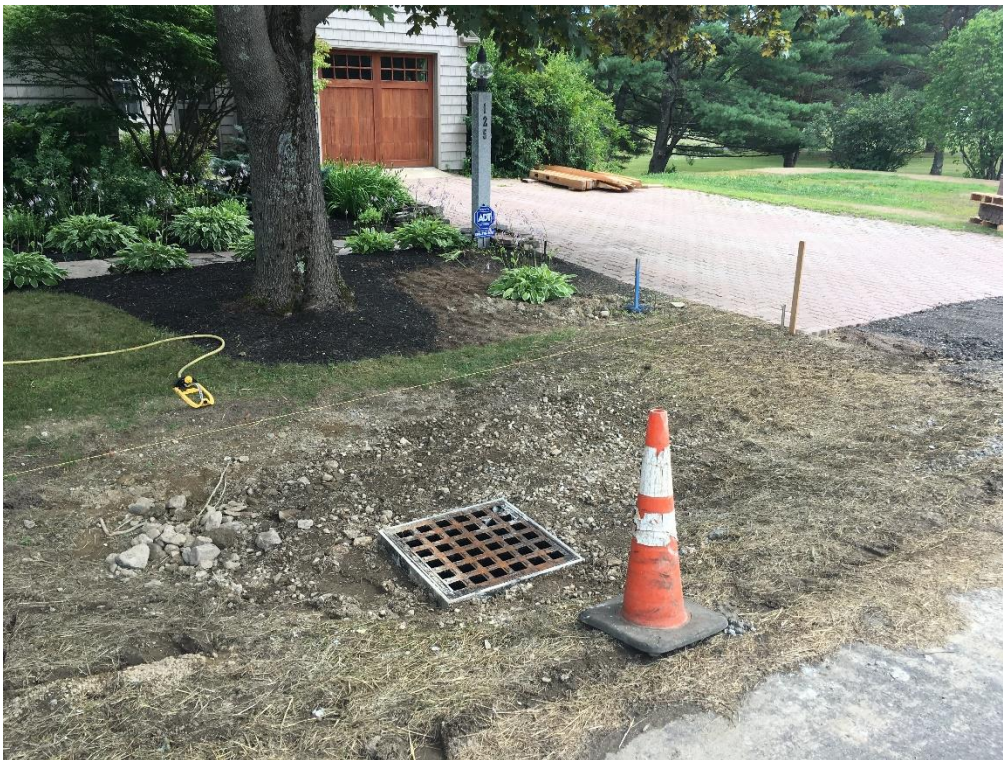
Storey Brothers installing frame & grates on catch basins and preparing driveways for pavement. CB-6E shown here in front of 125 Middle Road prior to placing loam & seed.
