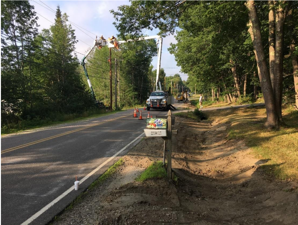
On Target started day transferring CMP wires just south of Range Way and north of Storey Brothers grubbing and excavating for drainage along the shoulder.
