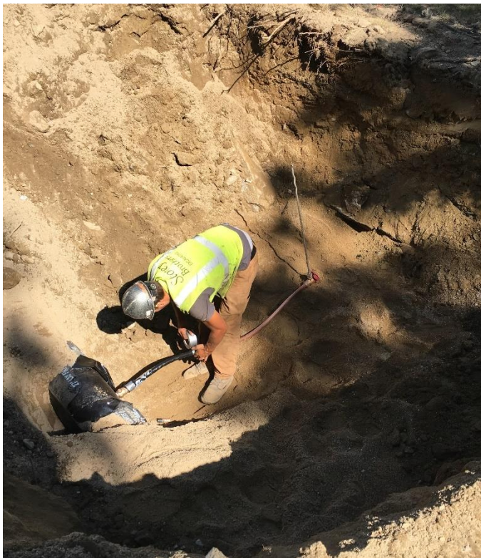
Installing water service from new water main extension to curb stop at 77 Middle Road.
