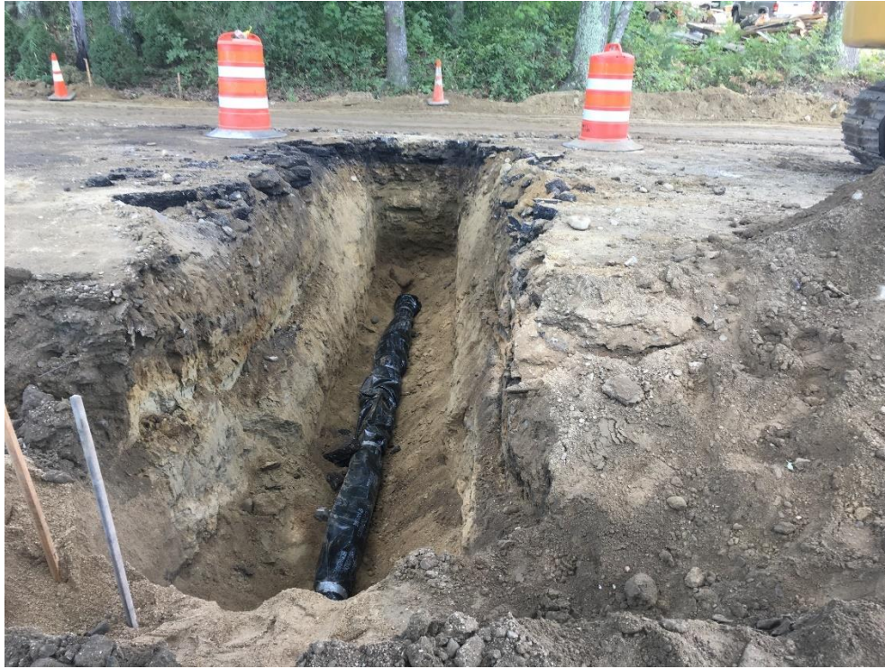
Trenching across road for hydrant at 76 Middle Road (STA 37+60).
