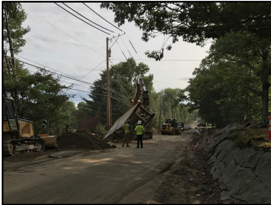
Photograph 4 - Friday, August 25 th – Removing Trench Box at STA 34+56
