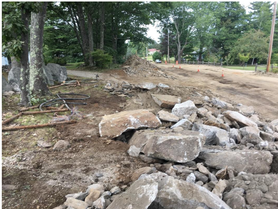
Photograph 10 - Wednesday, August 30 th – Ledge spoils from exposed bedrock outcropping in front of 70 to 72 Middle Road ready for removal.
