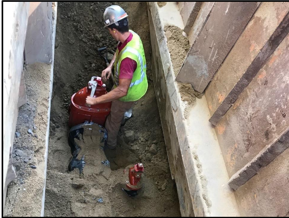
Photograph 1 – Thursday, August 24 th - Tee and Gate Valve for Hydrant at STA 37+60.
