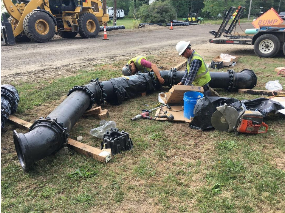
Photograph 7 – Tuesday, August 29 th – Assembling water main offset section to go under existing 24-inch culvert at STA 29+44.
