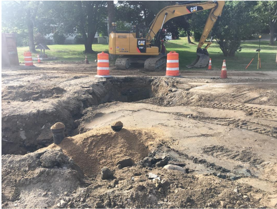
Photograph 9 – Wednesday, August 30 th – Trenching across road for hydrant at 54 Middle Road (STA 27+00).
