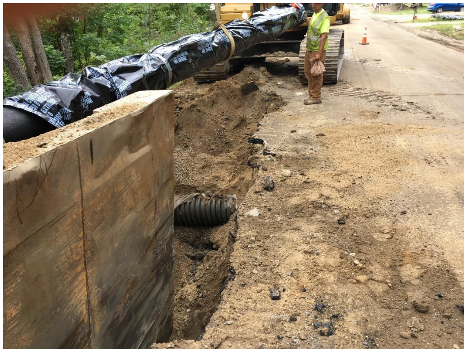
Photograph 8 - Tuesday, August 29 th – Placing a section of pipe prior to installing the offset section under culvert at STA 29+44.
