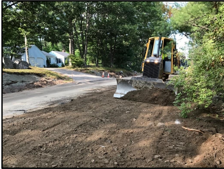
Photograph 3 – Friday, August 25 th - Backfill Water Line Trench at STA 35+00.
