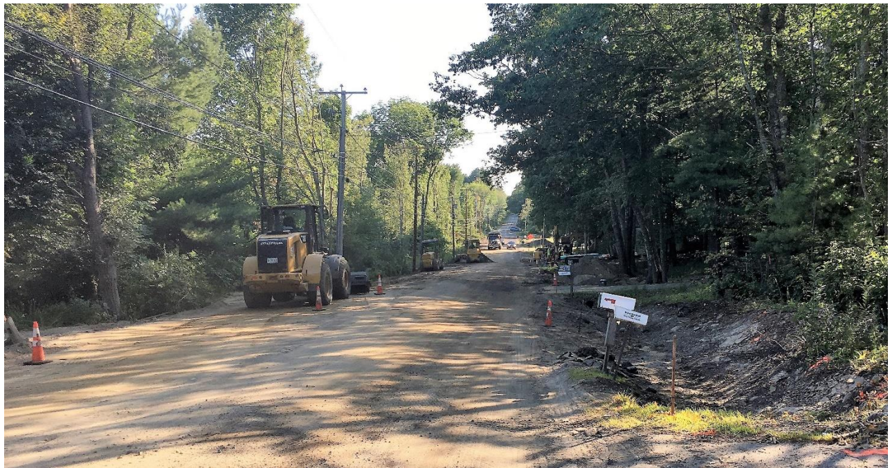
Photograph 6 - Monday, August 28 th – Backfilling after water main installation near STA 33+50
