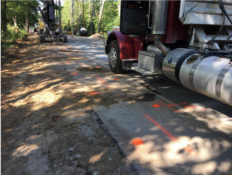
McGoldrick started drilling and blasting ledge for water main extension trench from STA 48+00 southward marking overburned depths every 10 feet.
