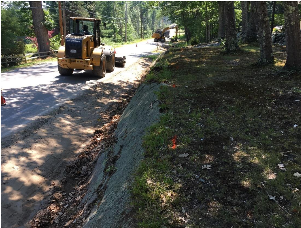
South of the pole work Storey Brothers proceeded southerly grubbing the sholders finishing up near Range Way approaching the southern end of the next phase of work. Ledge here at the backslope in front of 70 Middle Road.
