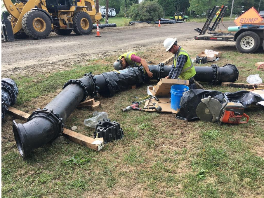
Assembling the water main section to go under the 24-inch culvert at STA 29+44.
