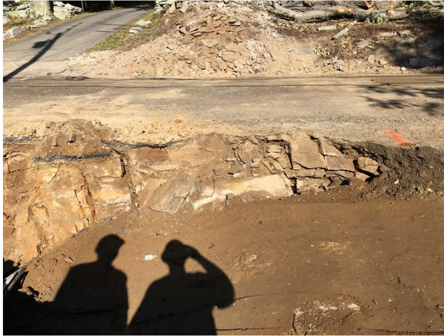
Extremely shallow ledge at STA 34+50.
