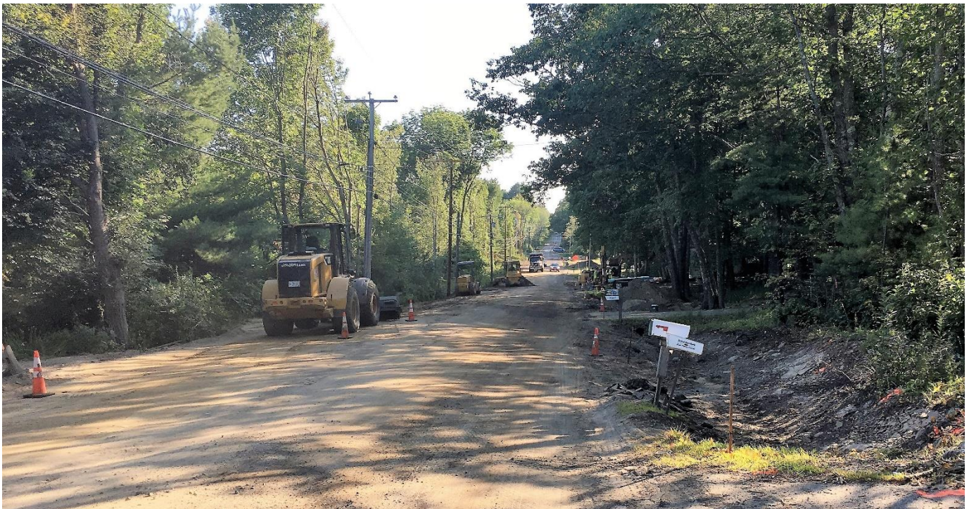
Backfilling after water main installation near STA 33+50.
