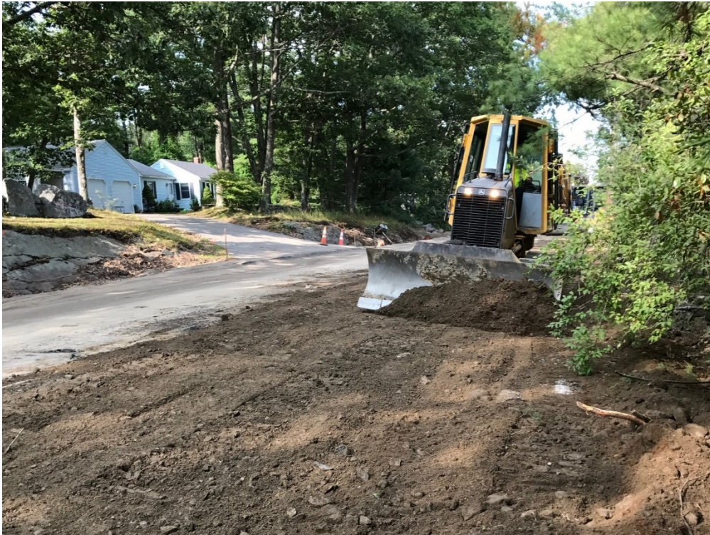
Backfill Water Line Trench at STA 35+00.
