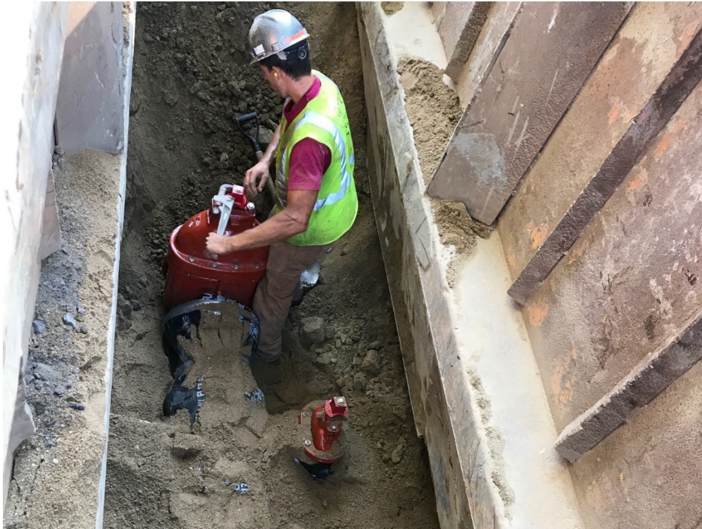
Tee and Gate Valve for Hydrant at STA 37+60.
