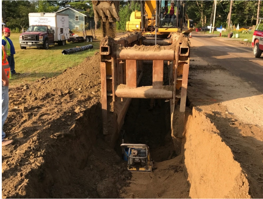
Water Main Installation, STA 40+60.
