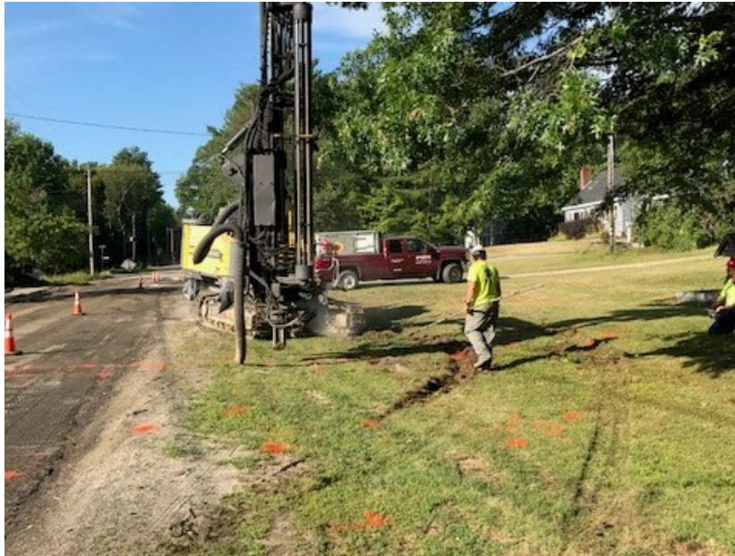
Photograph 9 – Wednesday, August 23 rd – Drilling and Blasting for Water Service Installation.
