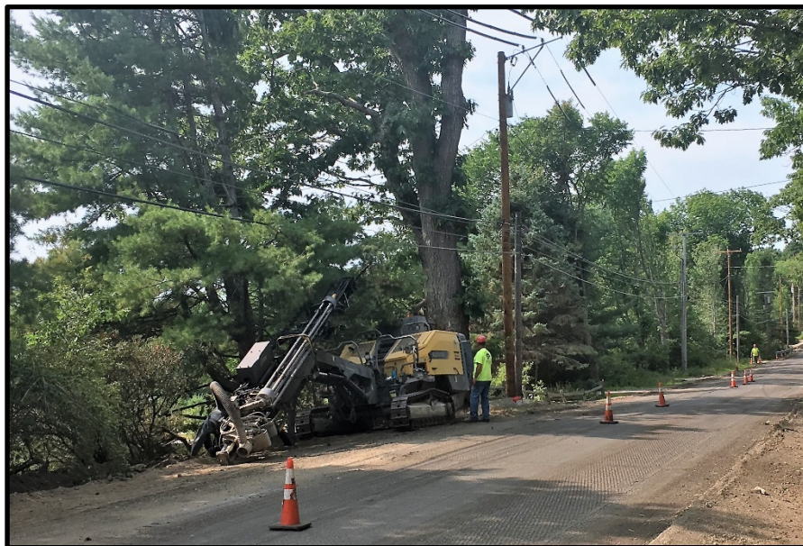
Photograph 2: Thursday, August 17 th - McGoldrick resumed drilling and blasting for the water main extension at 67 Middle Road southward.
