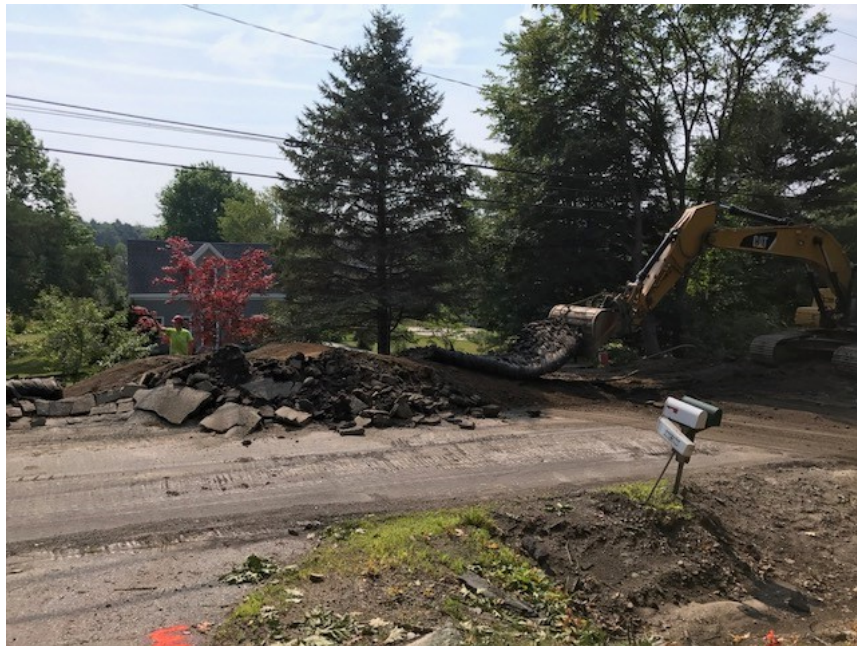
Photograph 6 - Monday, August 21 st – Blasting Ledge for Water Line Installation.
