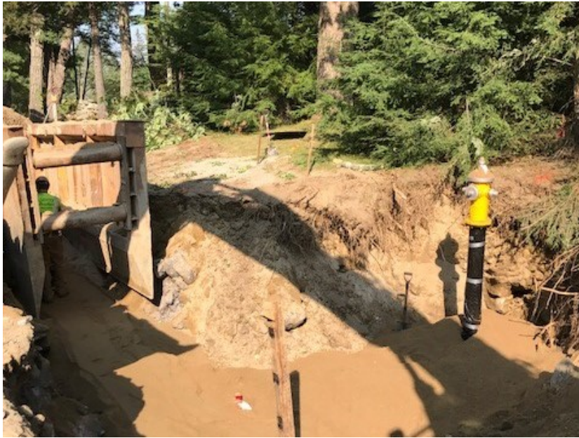
Photograph 7 – Tuesday, August 22 th – Hydrant and Air Valve Installation
