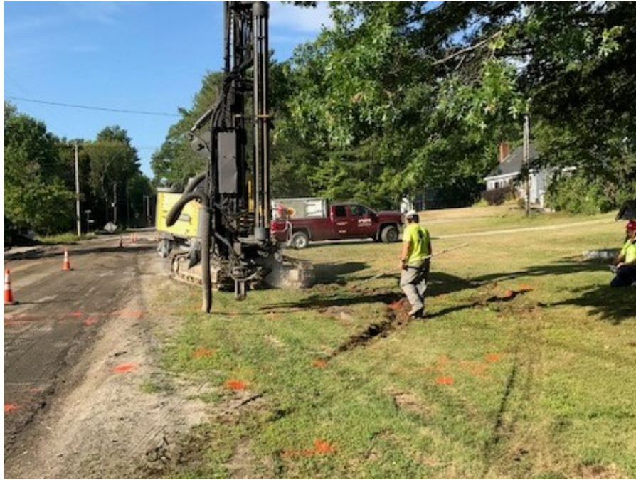
McGoldrick Drilling and Blasting for Water Service Installation.
