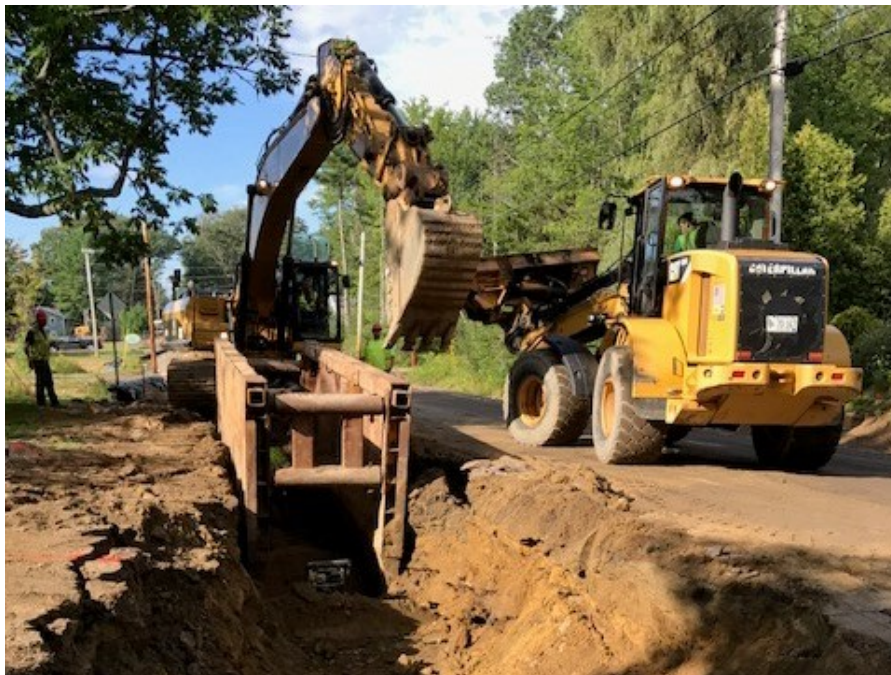
Water Main Installation, STA 44+00.
