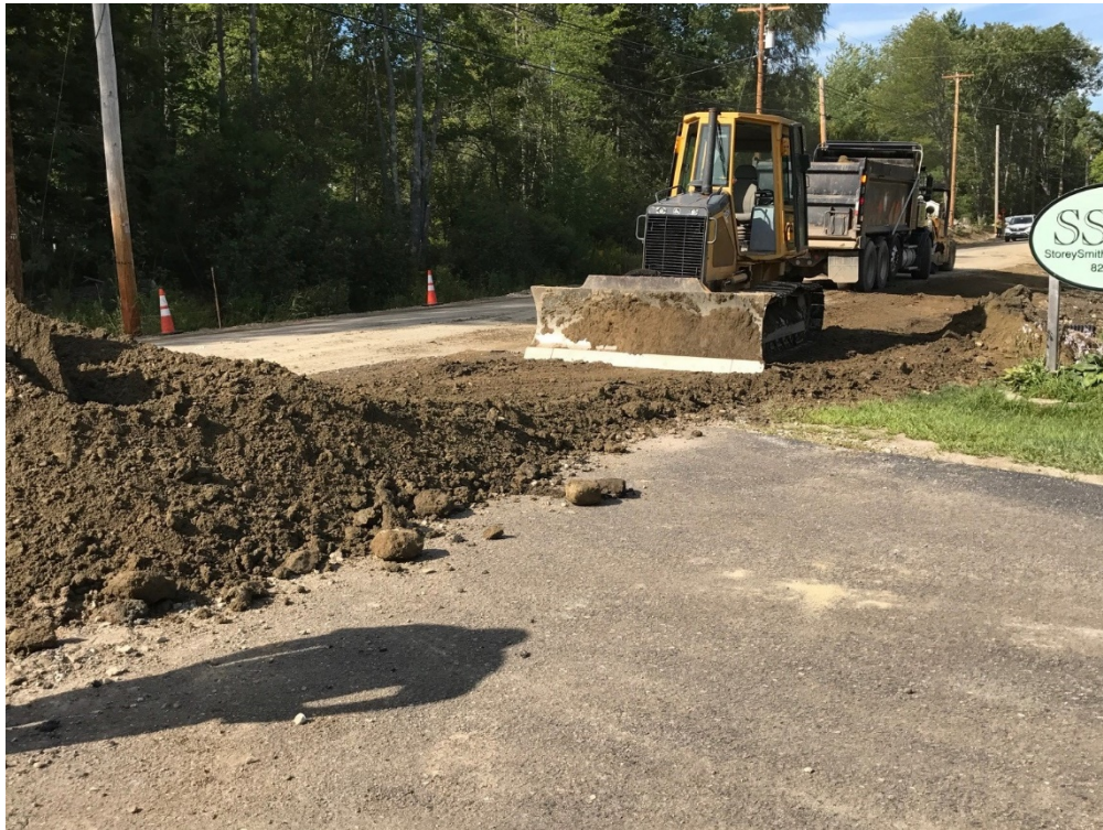
Backfill at Water Main Trench, STA 41+50
