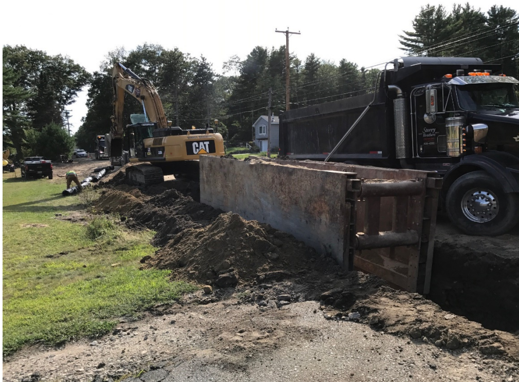
Water Main Installation, STA 41+00.
