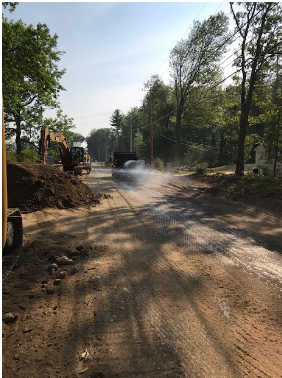
Watering Roadway for Dust Control
