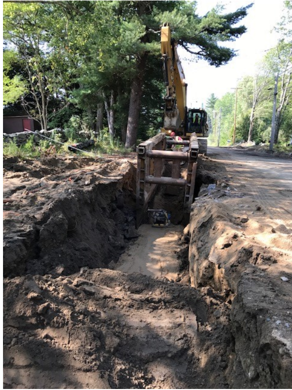
Water Line Installation STA 45+75.
