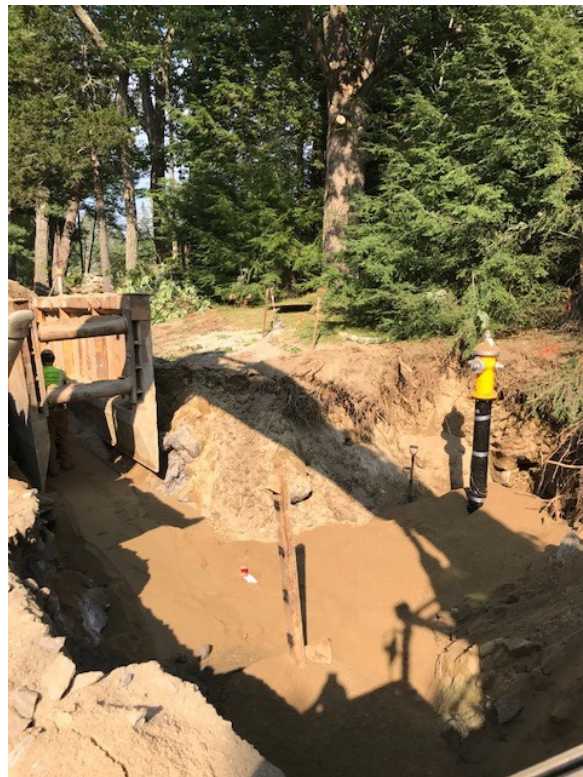
Hydrant Installation 44+87.
