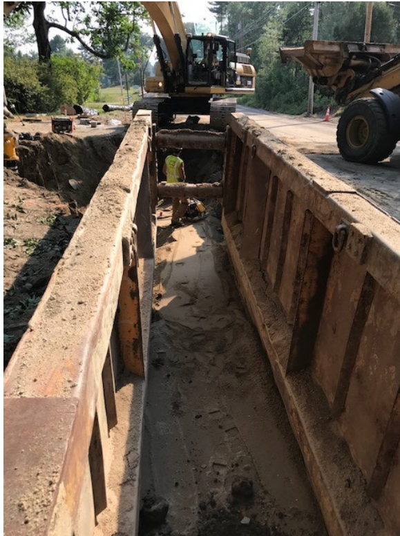
Compacting Sand Bedding, STA 44+75
