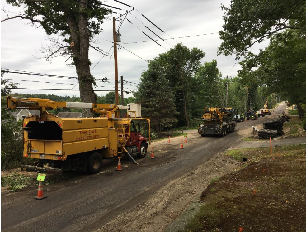
Placing crane and 2 bucket trucks for removal of large oak at 67 Middle Road. McGoldrick Brothers Blasting in background working away from the tree removal operation.
