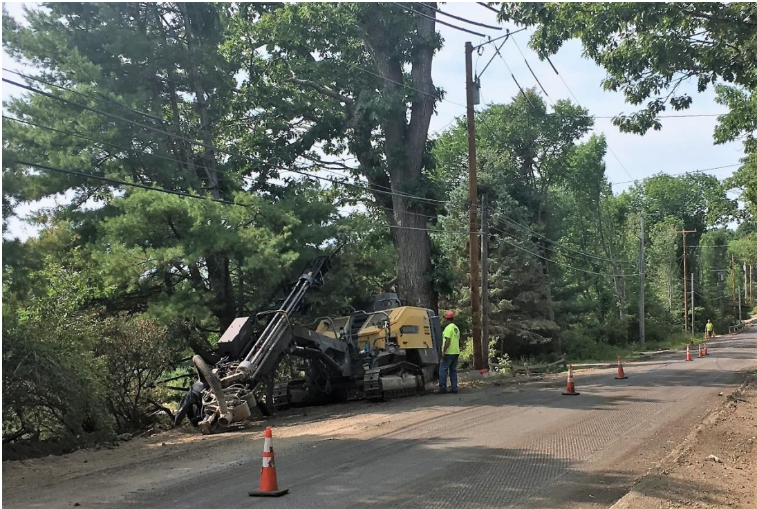
McGoldrick resumed drilling and blasting for the water main extension at 67 Middle Road southward.
