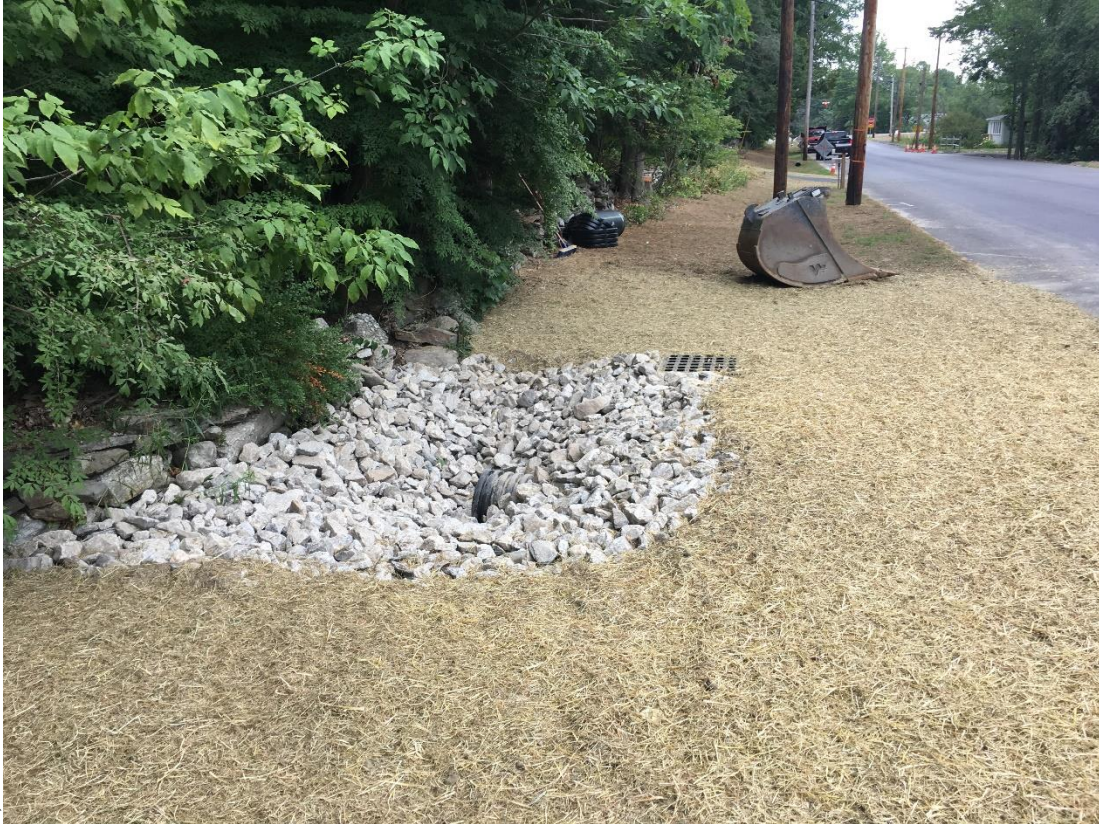
Installed a field inlet to the underdrain inlet pipe of CB-7E to pick up flow from an intermittent stream west of the rock wall. This catch basin had to be raised so outlet could clear water main.
