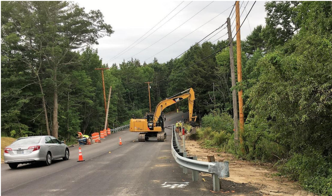
Removed the old guard rail on the inlet side of the Chenery Brook culvert. Cleared away weeds & small brush and leveled ground behind guardrail. Afterwards, placed loam, seed, & mulch.
