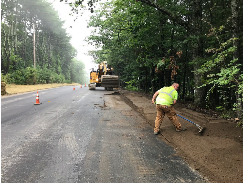
Photo 1 – Placing and raking topsoil near 3 Middle Road
