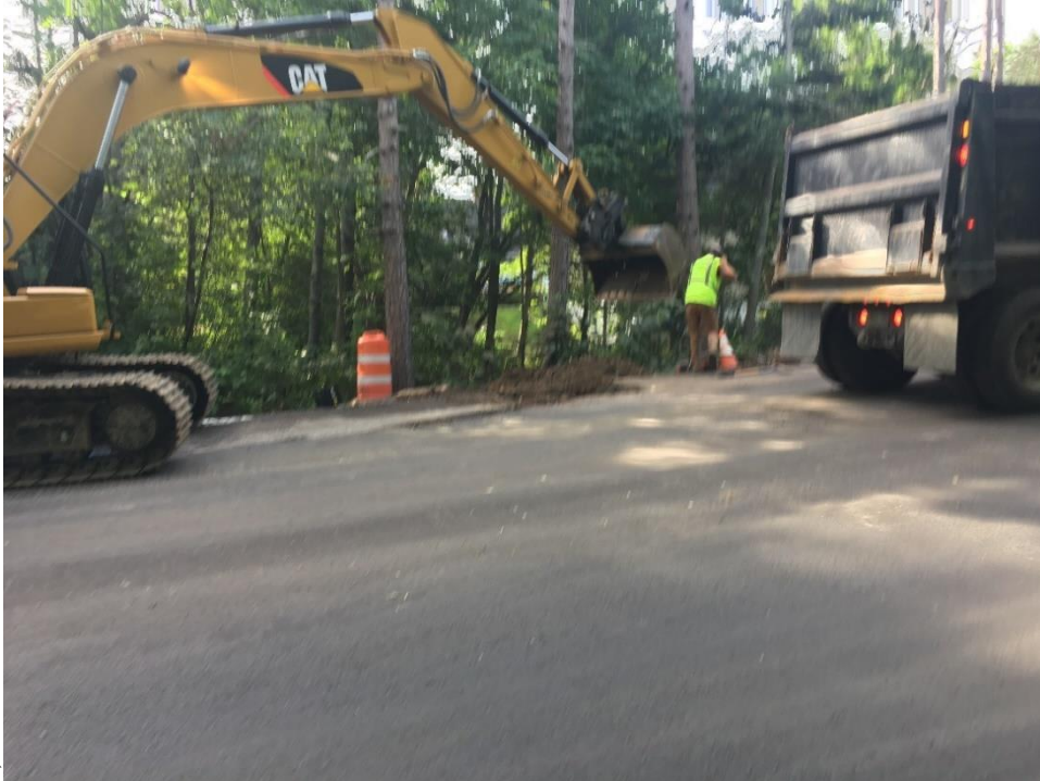
Saw cut around existing catch basin structures that were paved over in the gully section and then excavated to expose them to install frame & grate to new grade. Shown here is the existing catch basin at STA 52+00, Right.
