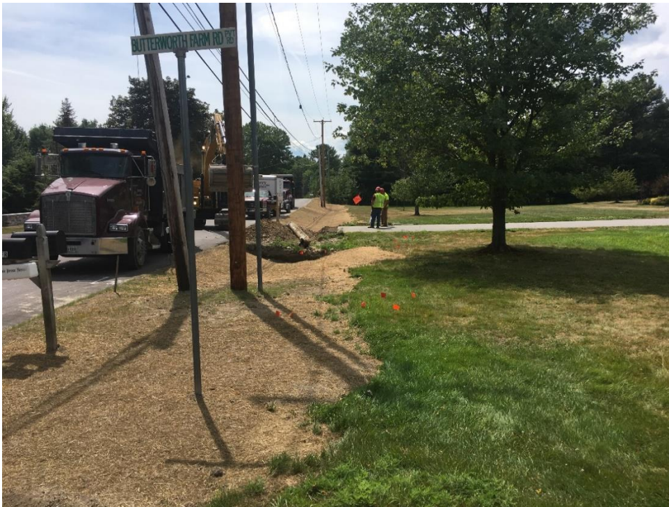
Installed new driveway culverts north of gully. Driveway for 126 Middle Road shown here at STA 65+00, Left.
