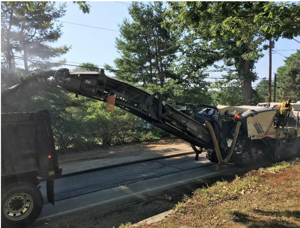
Milling shoulder of southbound lane in a northerly direction and conveying the millings onto trucks. These millings will be used later on the road as the top layer of gravel.
