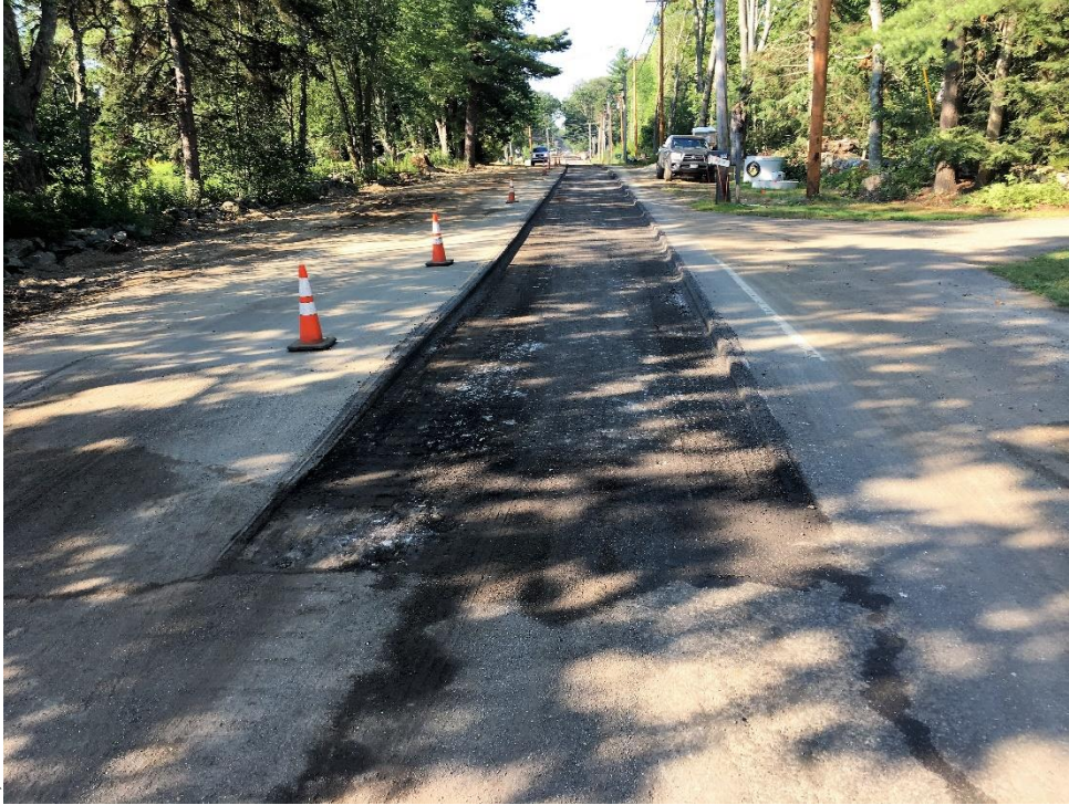
Beginning of 8'2' wide x 3 ½ inch deep pavement milling in southbound travel lane at STA 49+50 (near 95 middle Road) looking southward.
