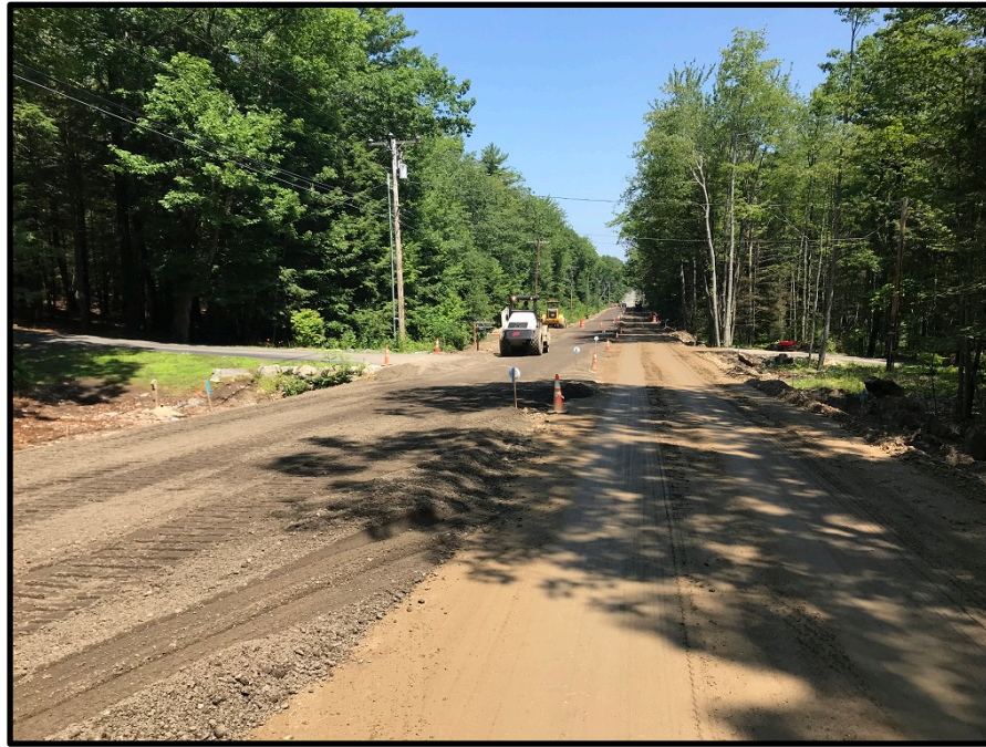
Photograph 3 - Friday , July 27 th – Compacting reclaim near 10 Middle Road
