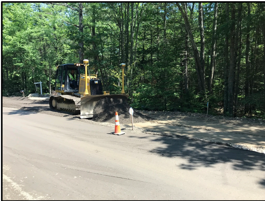
Photograph 4 - Friday, July 27 th – Grading reclaim near 23 Middle Road
