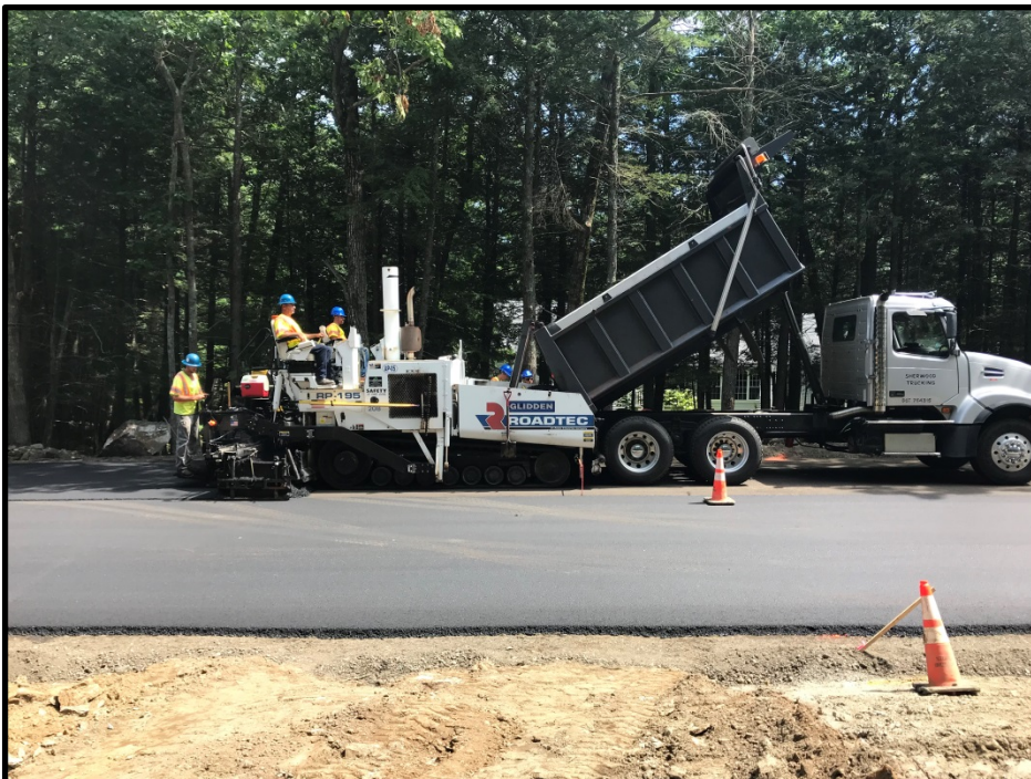
Photograph 8 - Tuesday, July 31 st – Paving east travel lane near Tall Pines Way
