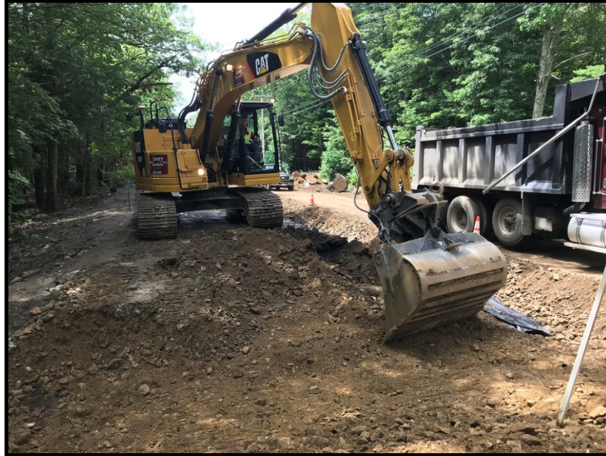
Photograph 1 – Thursday, July 26 th – Excavating to base grade at Tall Pines Way
