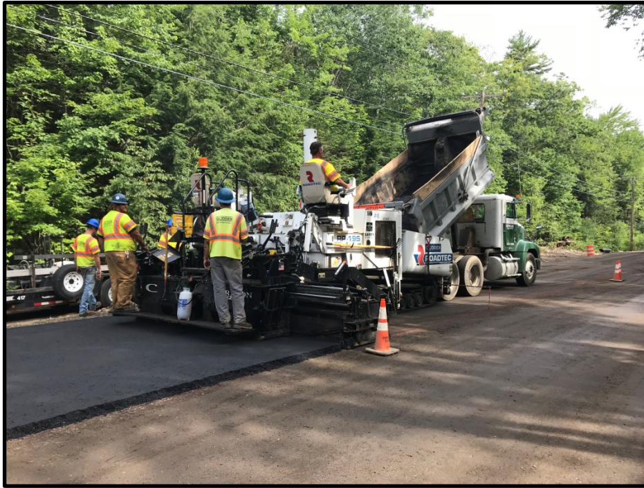
Photograph 7 – Tuesday, July 31 st – Paving west travel lane near existing bus turnaround
