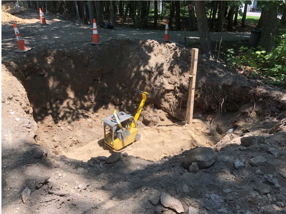
Photo 3 – Backfill water service at 10 Tall Pines Way
