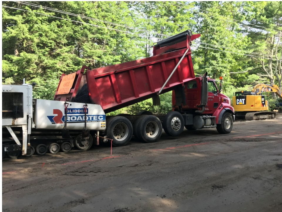
Photo 4 – Placing pavement in front of 4 Middle Road
