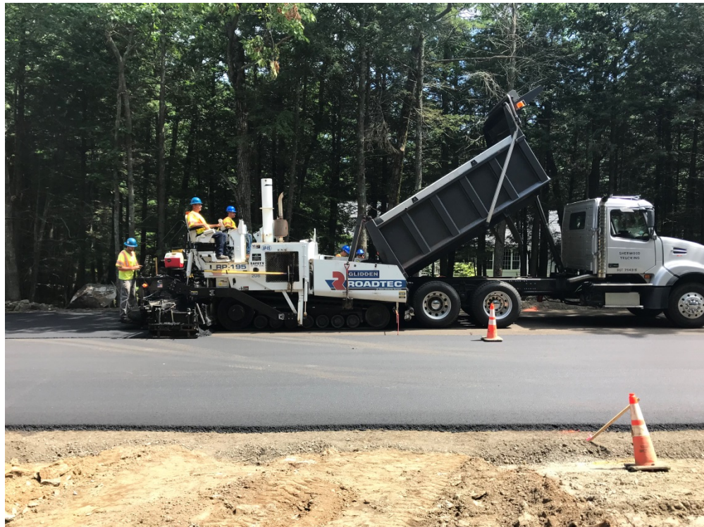
Photo 8 – Paving east site travel lane near Tall Pines Way
