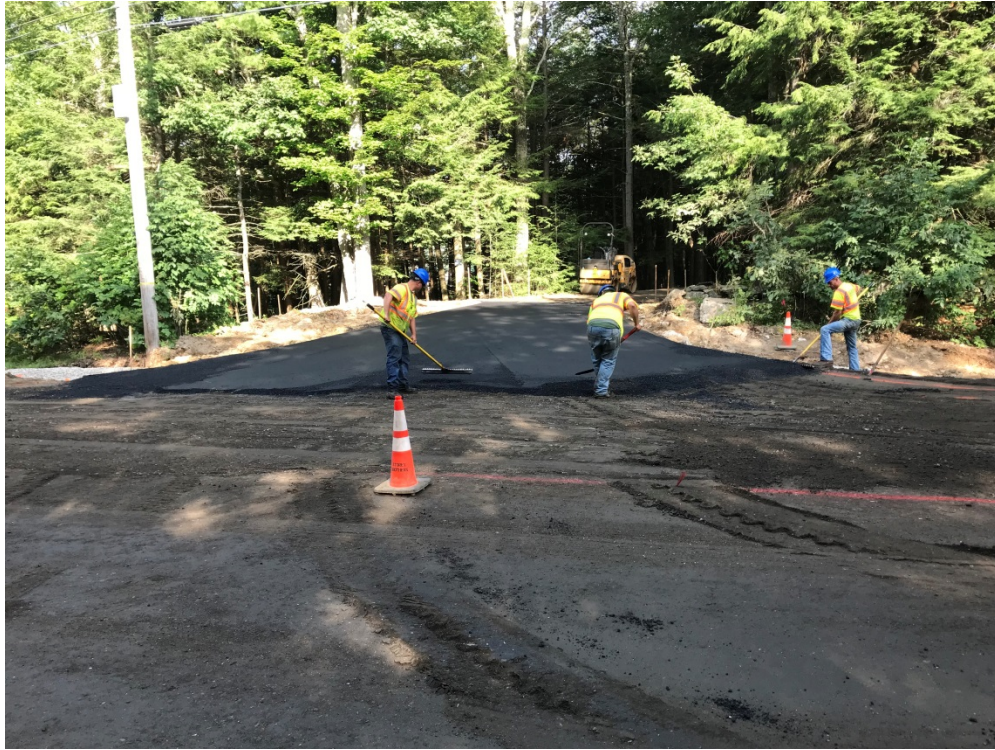
Photo 1 – Paving bus turnaround at 4 Middle Road
