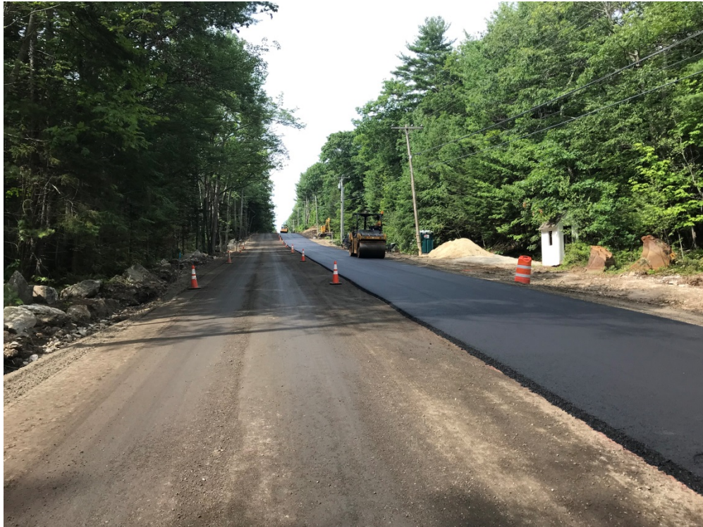
Photo 6 – Compacting pavement
