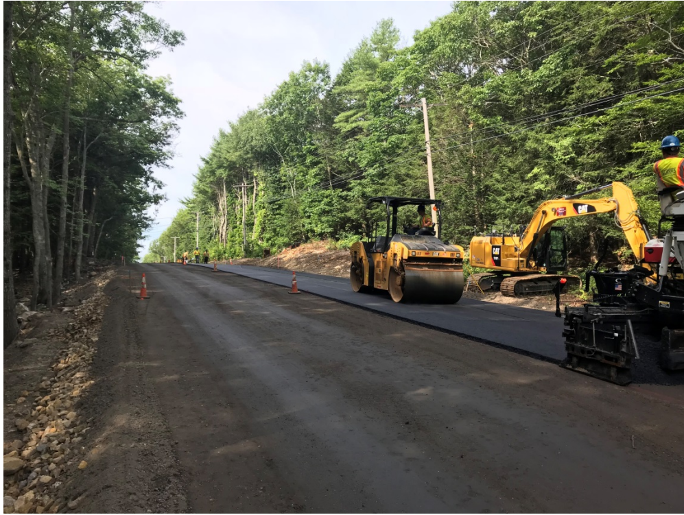
Photo 5 – Compacting pavement
