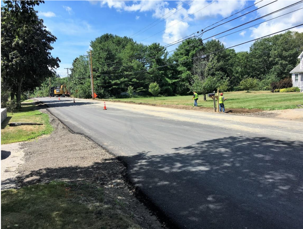
Shaping swale and placing loam southerly from Butterworth Farm Road along the west side of road in front of 126 Middle Road.
