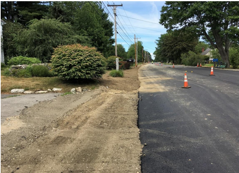
Southern extent of loam & seed at STA 61+10 (Eddy driveway at 122 Middle Road) prior to the placement of straw mulch at the end of the day.
