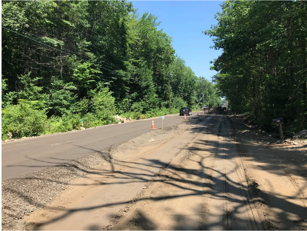
Photo 1 – Placing reclaim base to prep for pavement
