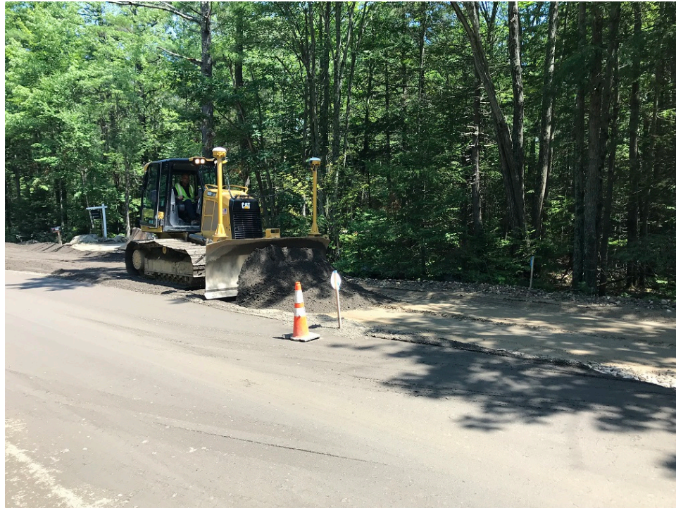
Photo 4 – Grading reclaim near 23 Middle Road
