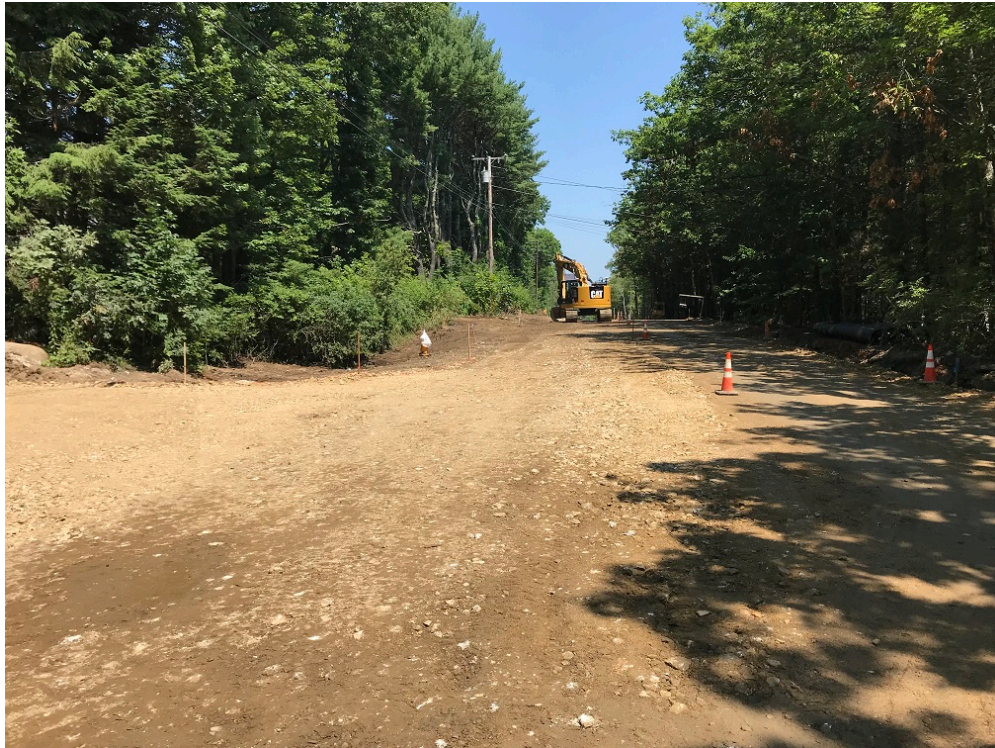
Photo 2 – Grading side slopes off edge of road
