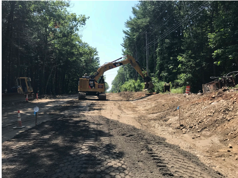
Photo 6 – Grading side slopes in front of 4 Middle Road
