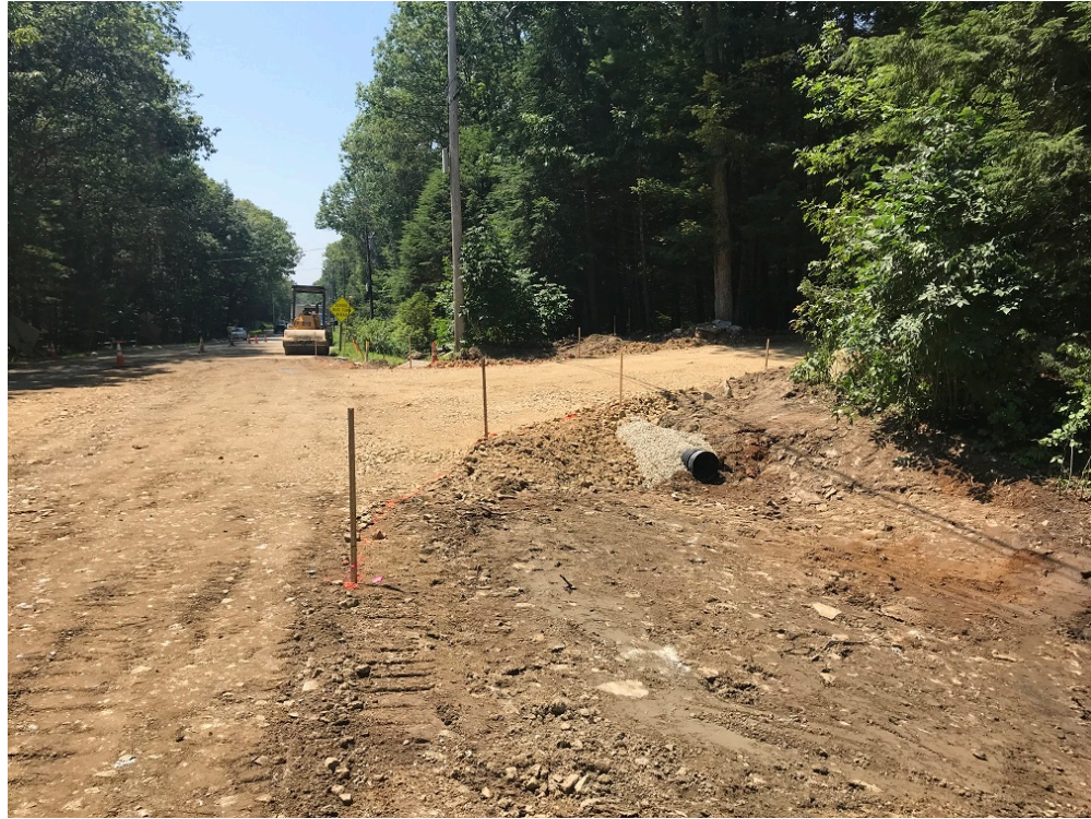
Photo 3 – Installed culvert and graded bust turnaround at 4 Middle Road
