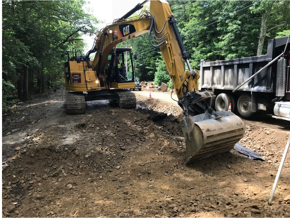
Photo 3 – Excavating for base grade
