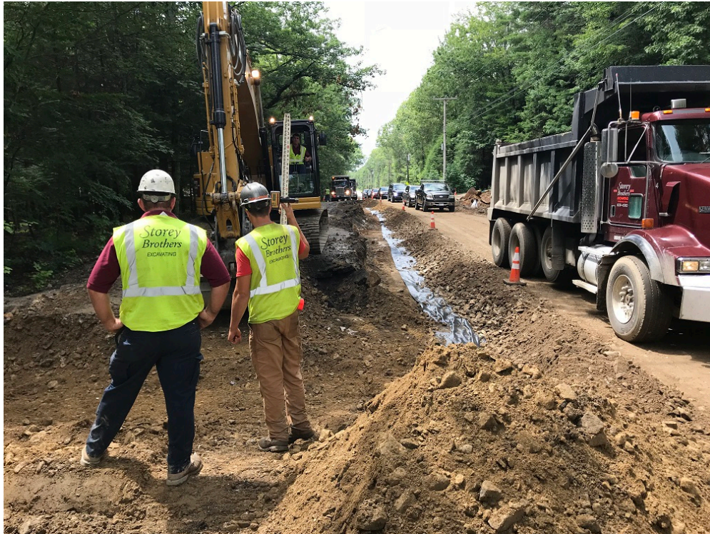
Photo 2 – Checking base grade near Tall Pines Way
