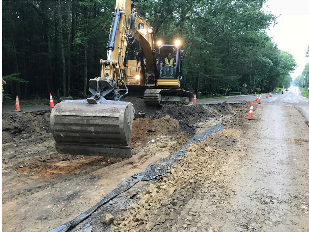
Photo 7 – Excavating for box cut near Falmouth Town Line
