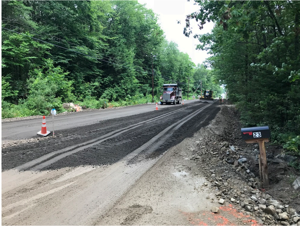
Photo 1 – Placing base gravel near Evergreen Lane
