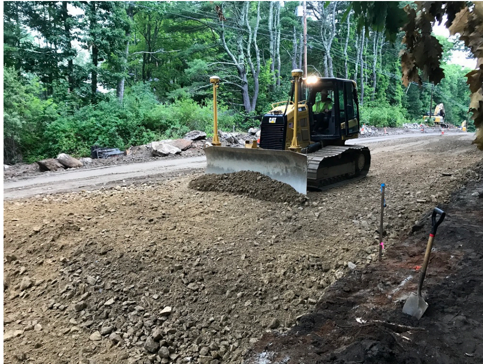
Photo 4 – Grading subbase gravel near Falmouth Town Line
