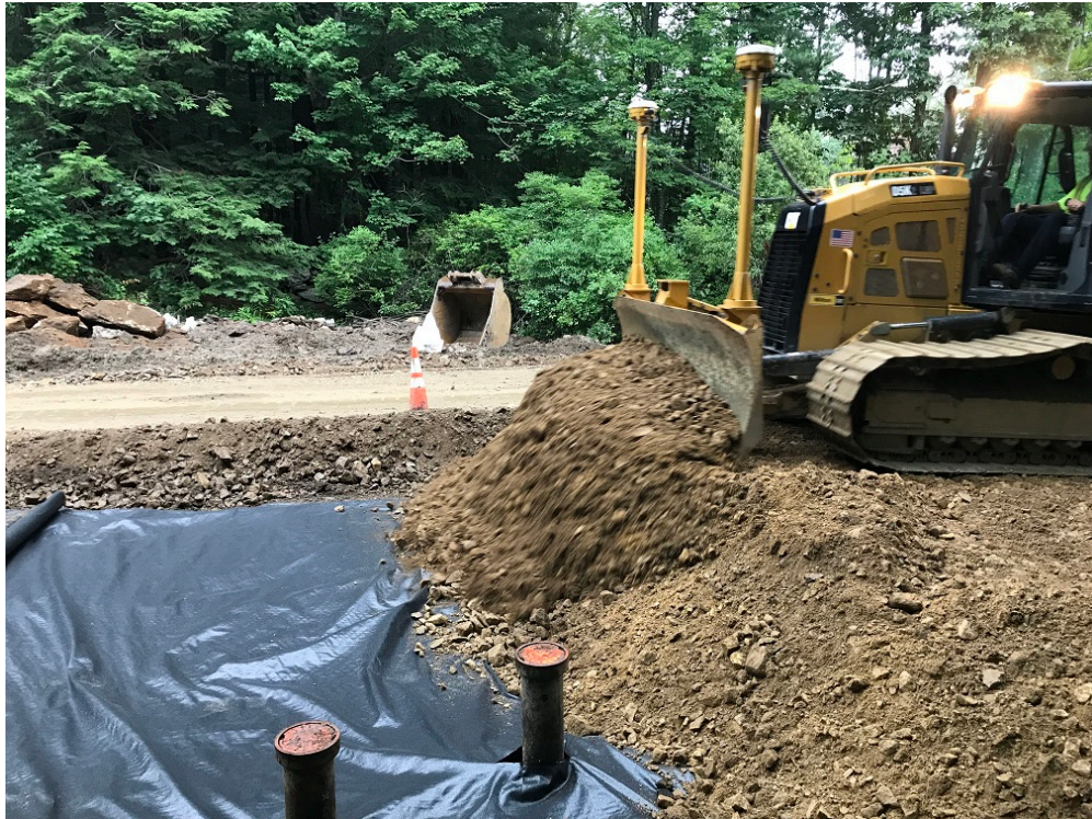
Photo 6 – Placing subbase gravel near Falmouth Town Line
