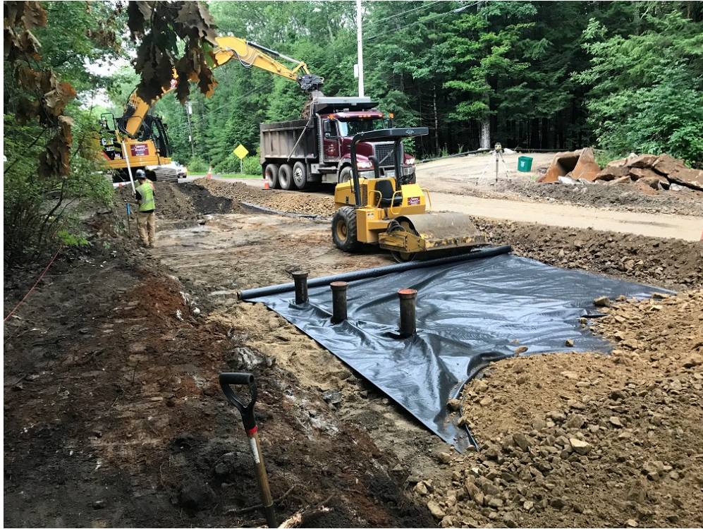
Photo 5 – Compacting base near Falmouth Town Line
