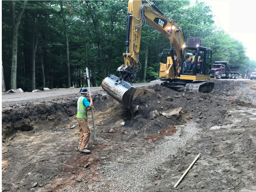
Photo 3 – Excavating for base grade near Tall Pines Way
