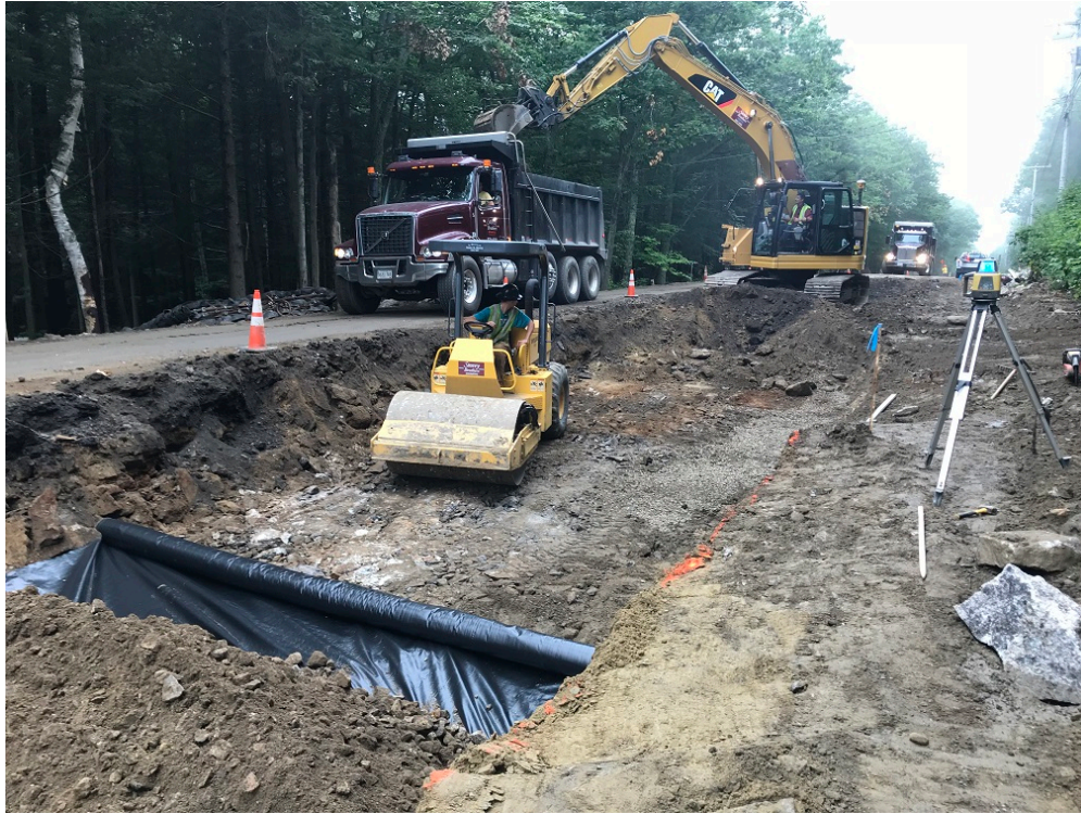
Photo 1 – Excavating for base grade near Tall Pines Way
