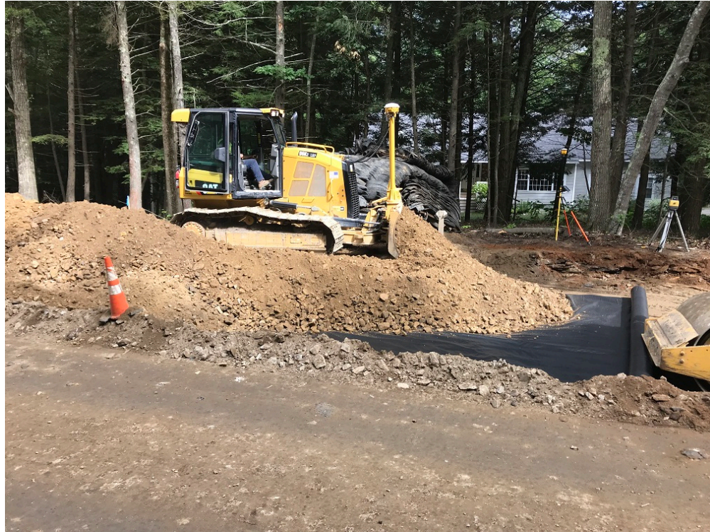
Photo 7 – Grading subbase gravel
