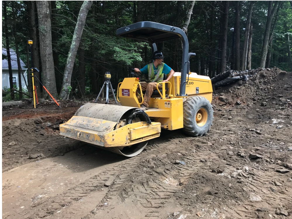
Photo 6 – Compacting the base
