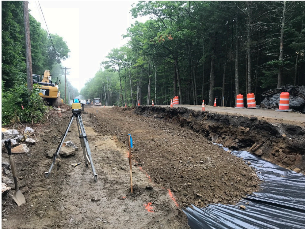
Photo 2 – Subbase gravel placement near Tall Pines Way
