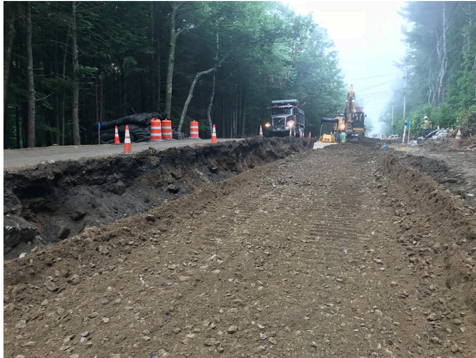
Photo 4 – Placing subbase gravel
