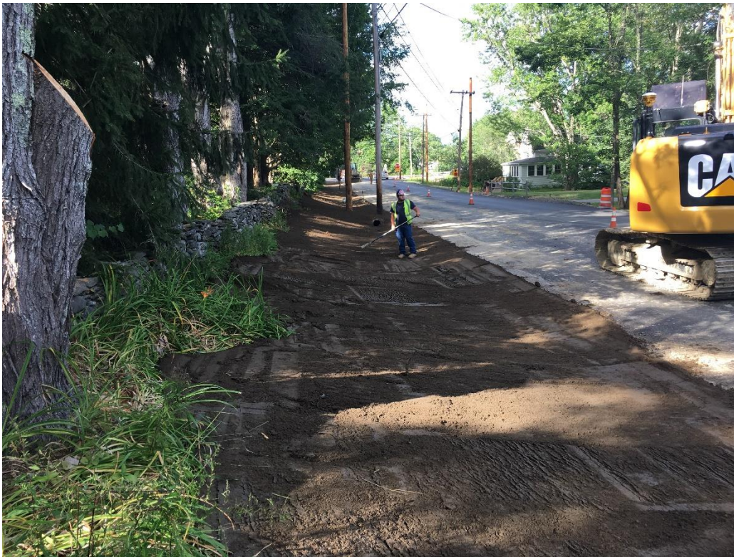
Performed preliminary finish work to previously paved section by placing loam and seed.
