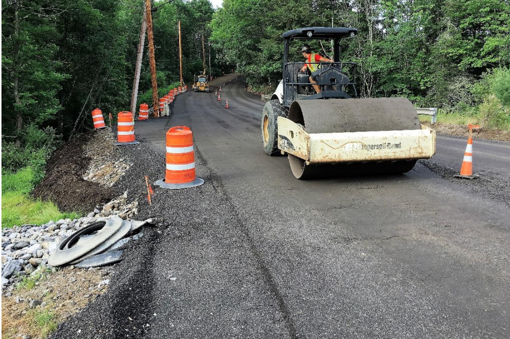
Began the day placing and compacting screened pavement millings over Type D subbase gravel in northbound lane from STA 55+80 southward to STA 48+50.
