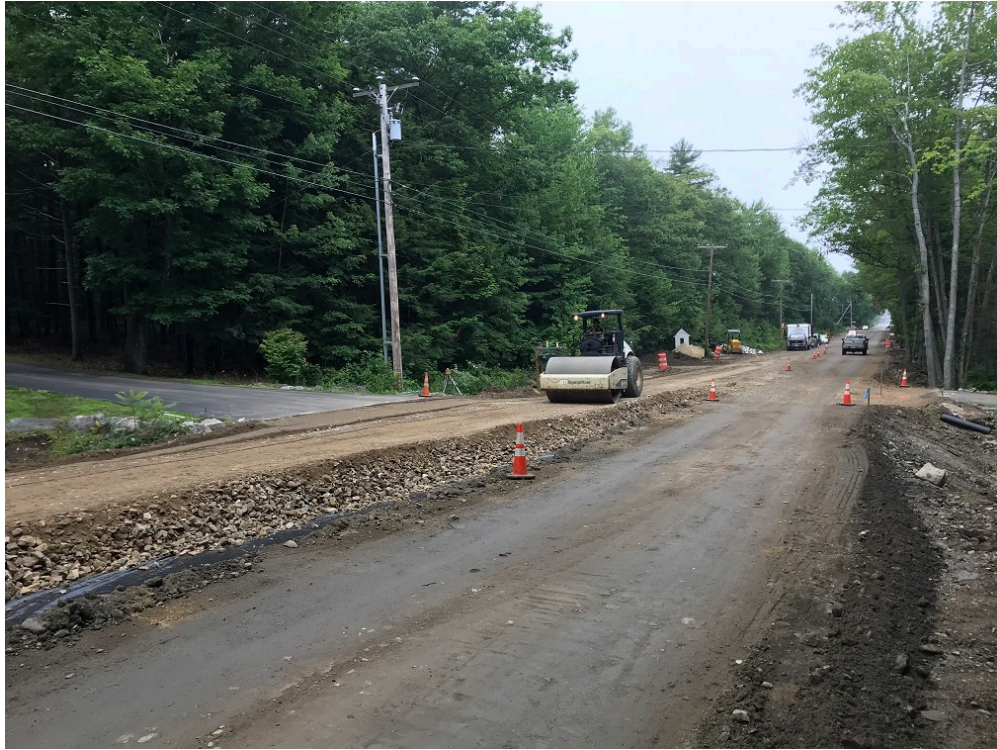
Photo 3 – Compacting subbase gravel in front of 10 Middle Road
