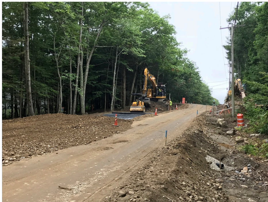
Photo 8 – Excavating for gravel placement
