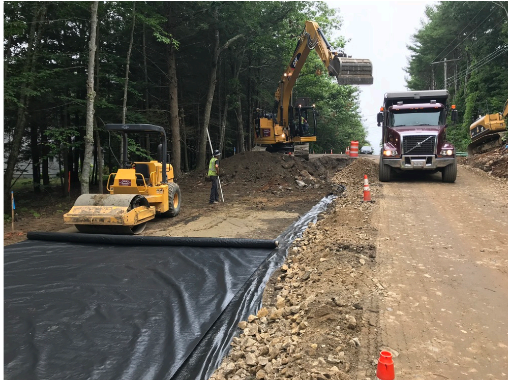
Photo 6 – Checking base grade and placing fabric
