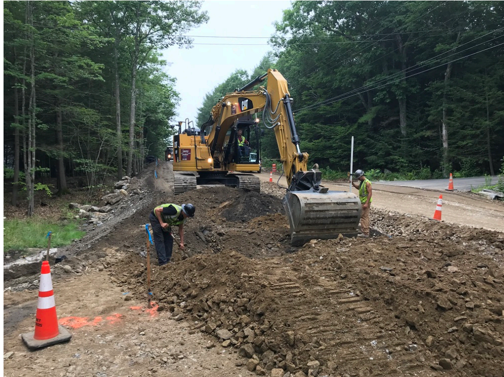
Photo 5 – Excavating to base grade near 15 Middle Road
