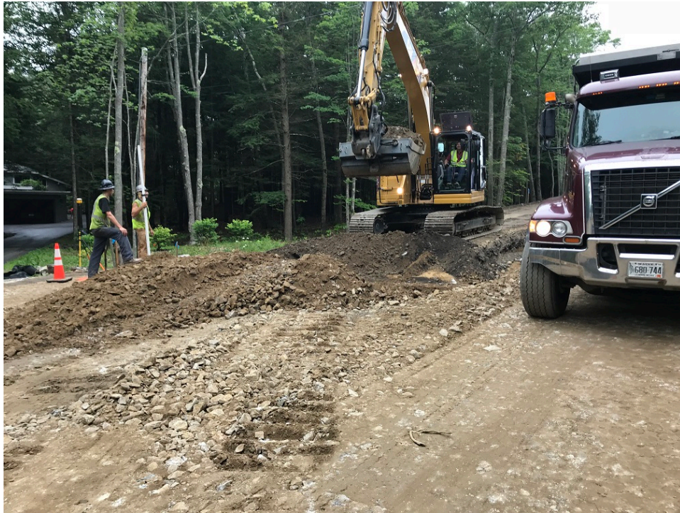
Photo 4 – Excavating to base grade near 15 Middle Road
