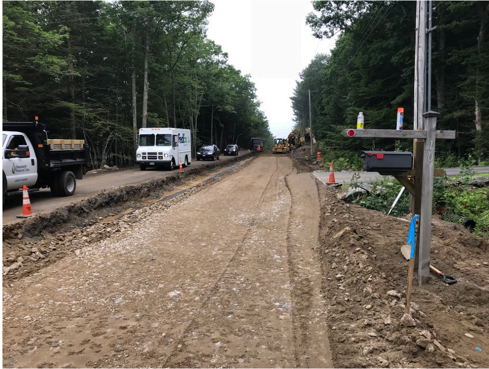
Photo 1 – Placing and compacting subbase gravel
