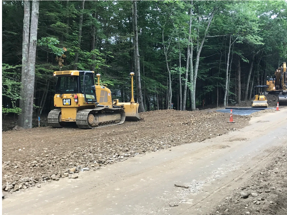
Photo 7 – Grading subbase gravel
