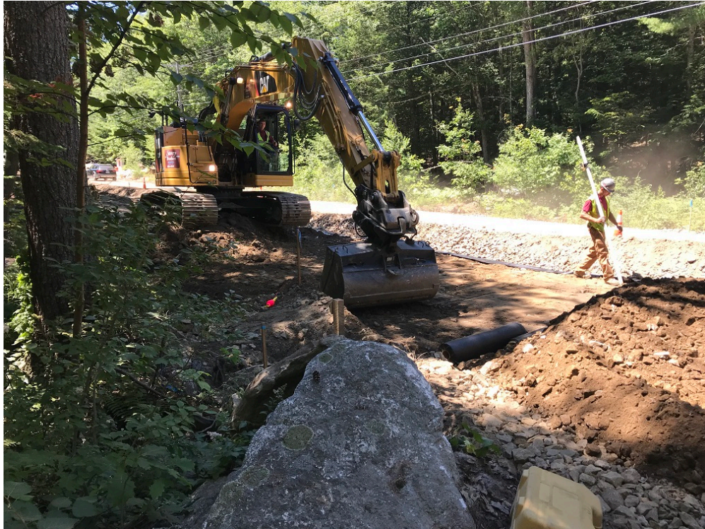
Photo 5 – Checking base grade for full depth construction
