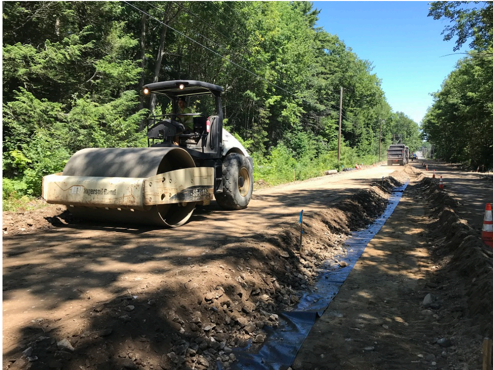
Photo 2 – Compacting subbase gravel
