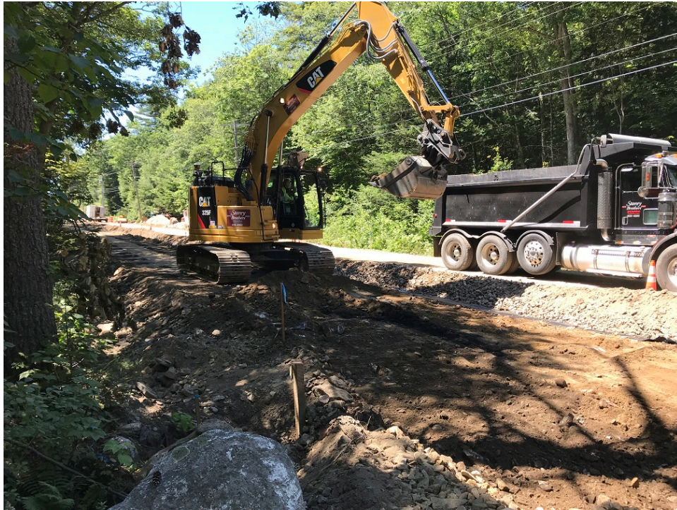
Photo 4 – Excavating to base grade on east side of Middle Road
