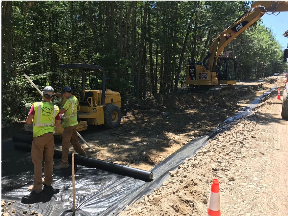
Photo 8 – Excavating for full depth road reconstruction
