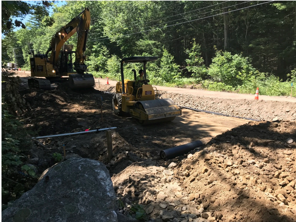
Photo 6 – Compacting base material
