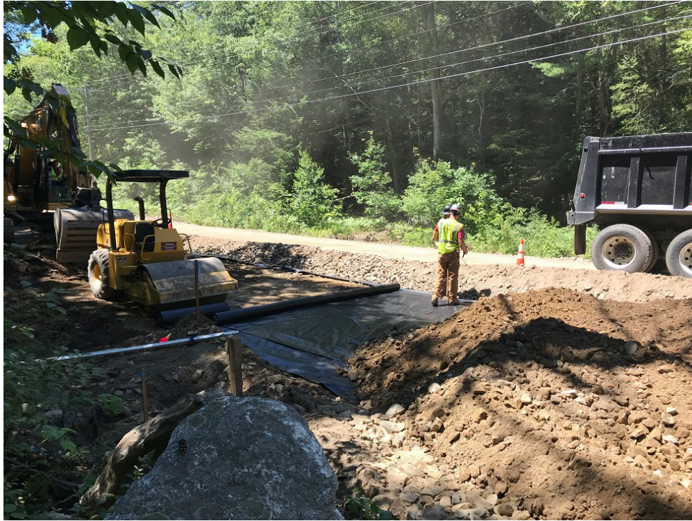
Photo 7 – Placing fabric over base grade before gravel placement
