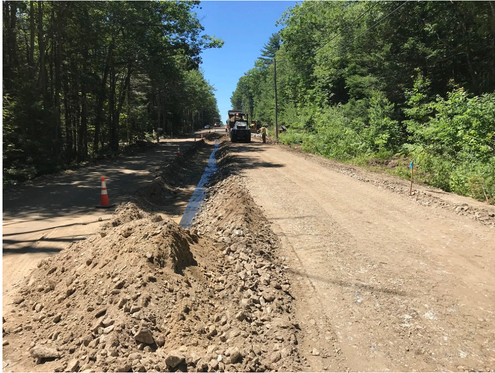
Photo 1 – Compacting subbase gravel near STA 8+00
