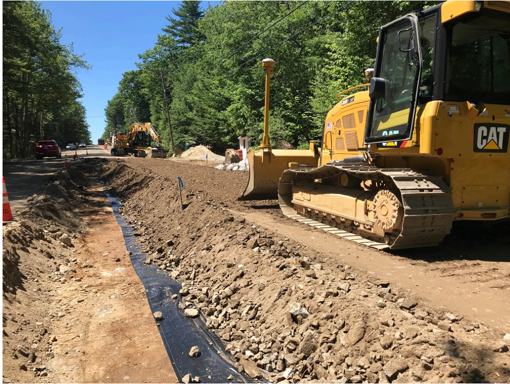
Photo 3 – Grading subbase gravel near existing bus turnaround
