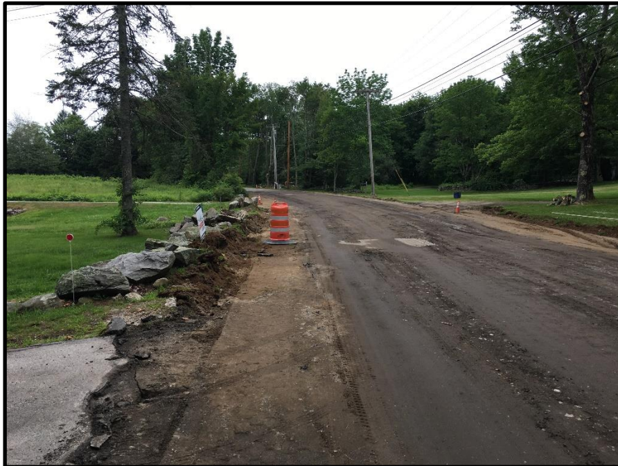
Photograph 2: Thursday, July 13 th - Finished pavement removal and grubbing on the eastern side of road by the end of the day.
