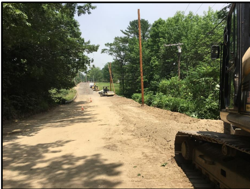
Photograph 10 - Wednesday, July 19 th - Placement and compact of gravel along eastern shoulder through the “Chernery Brook Gully.”
