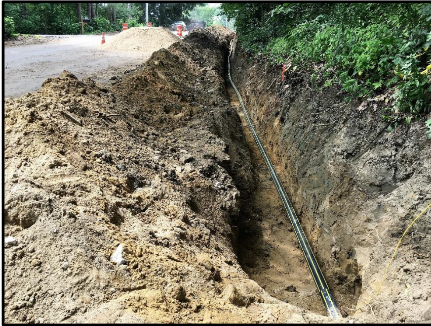
Photograph 7 – Tuesday, July 18 th - Mid-day placement of gas line from end of previous day's installation looking south
