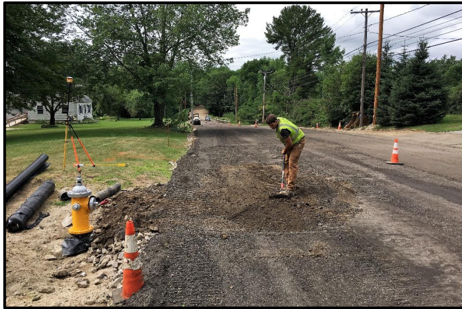
Photograph 3 – Friday, July 14 th - Installing new valve box prior to re-compaction.
