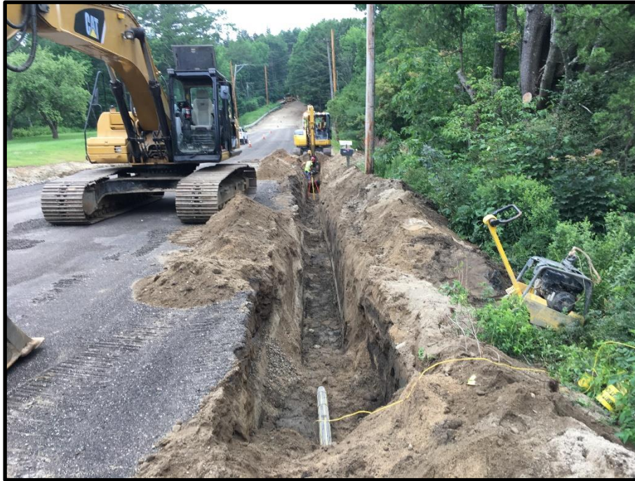
Photograph 5 – Monday, July 17 th – Exposing the previously installed gas main and excavating along the western edge of road southward approaching the Chernery Brook Gully.
