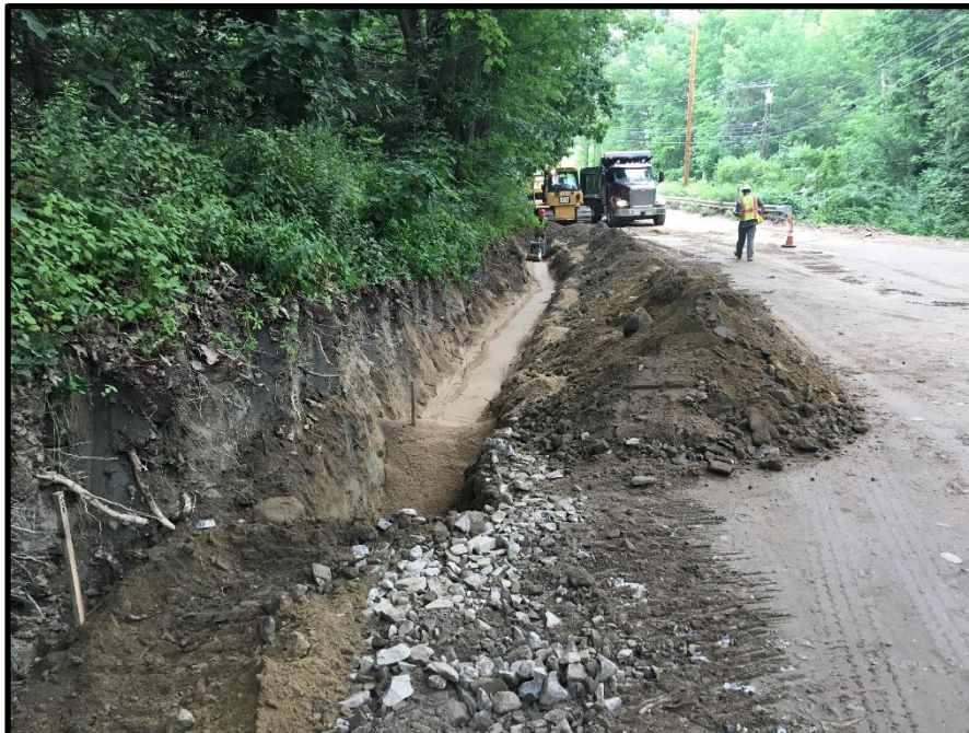
Photograph 6 - Monday, July 17th - Finishing up 640 linear feet of gas main installation near the end of the day south of Chernery Brook at STA 53+00.
