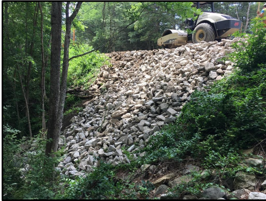
Photograph 9 – Wednesday, July 19 th - Placement of “Heavy Rip Rap” on outlet side of Chernery Brook Gully above outlet of 42-inch culvert at STA 55+80.
