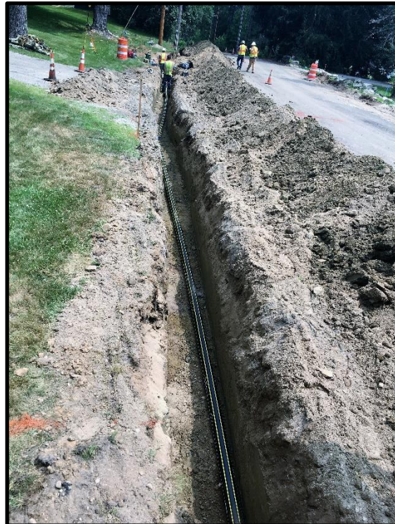
Photograph 8 - Tuesday, July 18 th - Looking back from the southern limit of progress prior to fusing pipe and backfilling.
