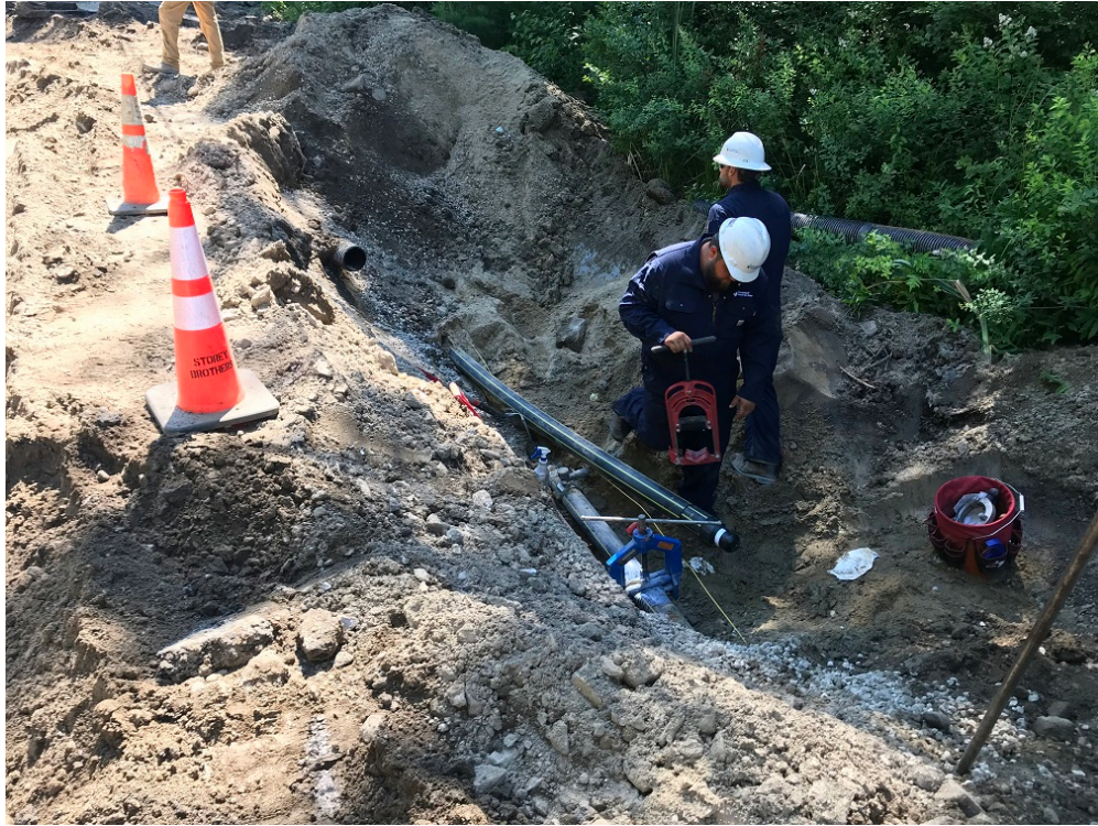
Photo 7 – Making gas main connection with work completed in 2017
