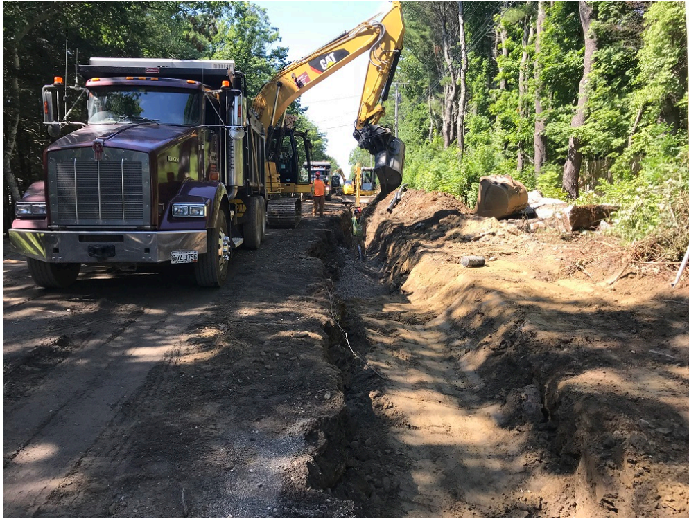
Photo 1 – Placing stone on 4 inch underdrain in front of 4 Middle Road
