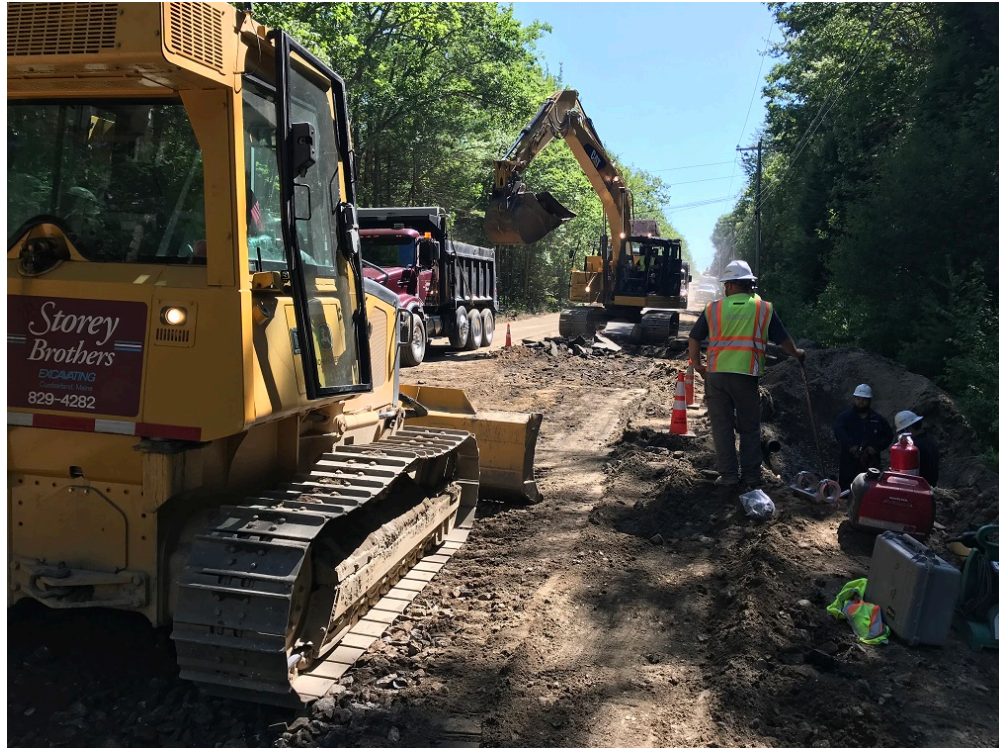
Photo 6 – Removing pavement for full depth road construction south of Evergreen Lane
