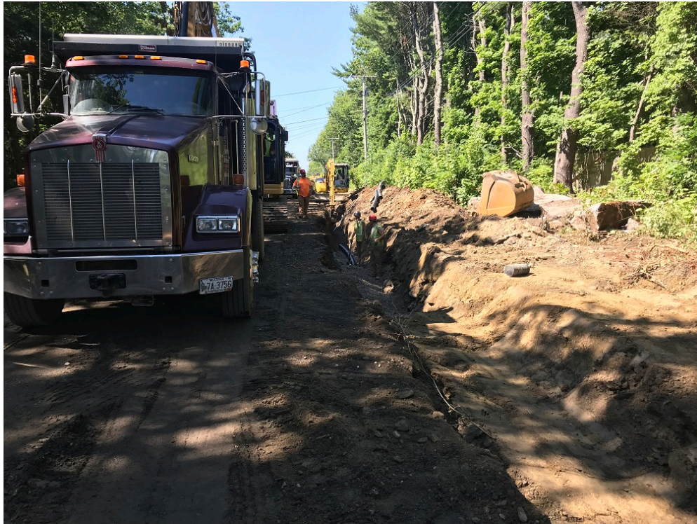
Photo 2 – Installing 4 inch underdrain in front of 4 Middle Road
