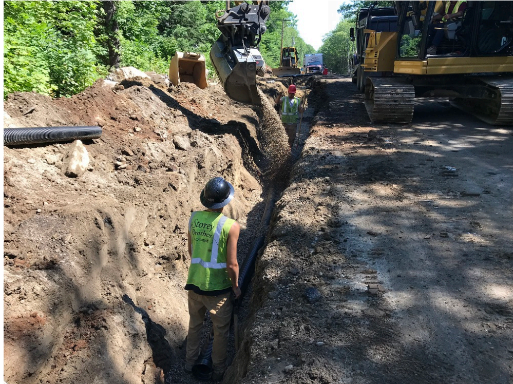
Photo 5 – Placing stone over 4 inch underdrain
