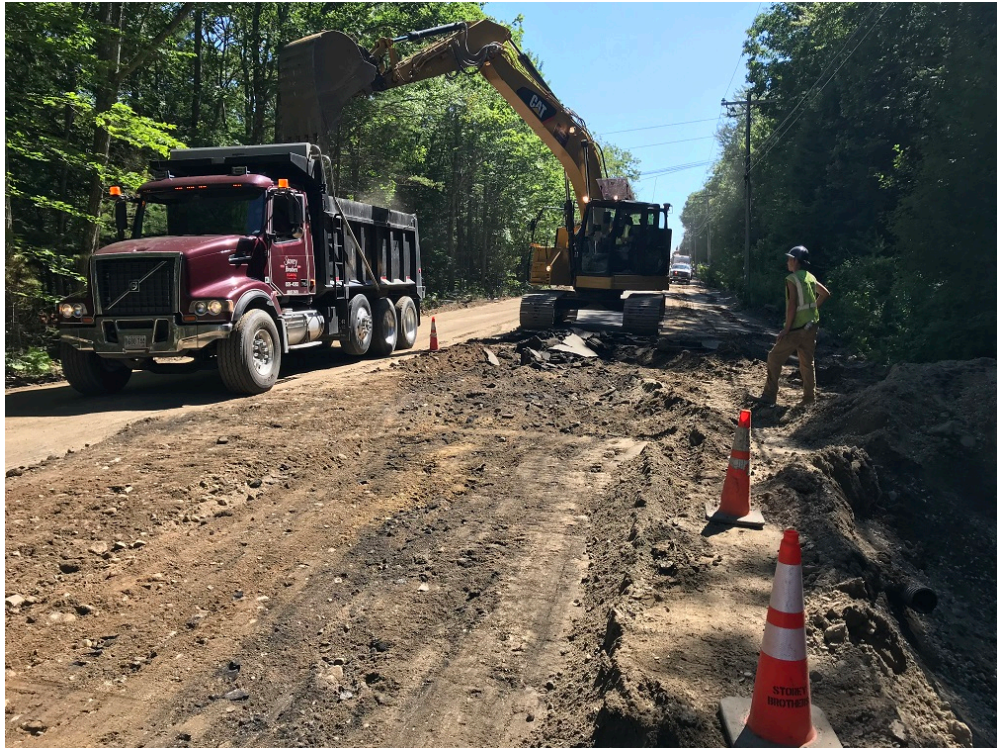
Photo 8 – Removing pavement for full depth road construction south of Evergreen Lane
