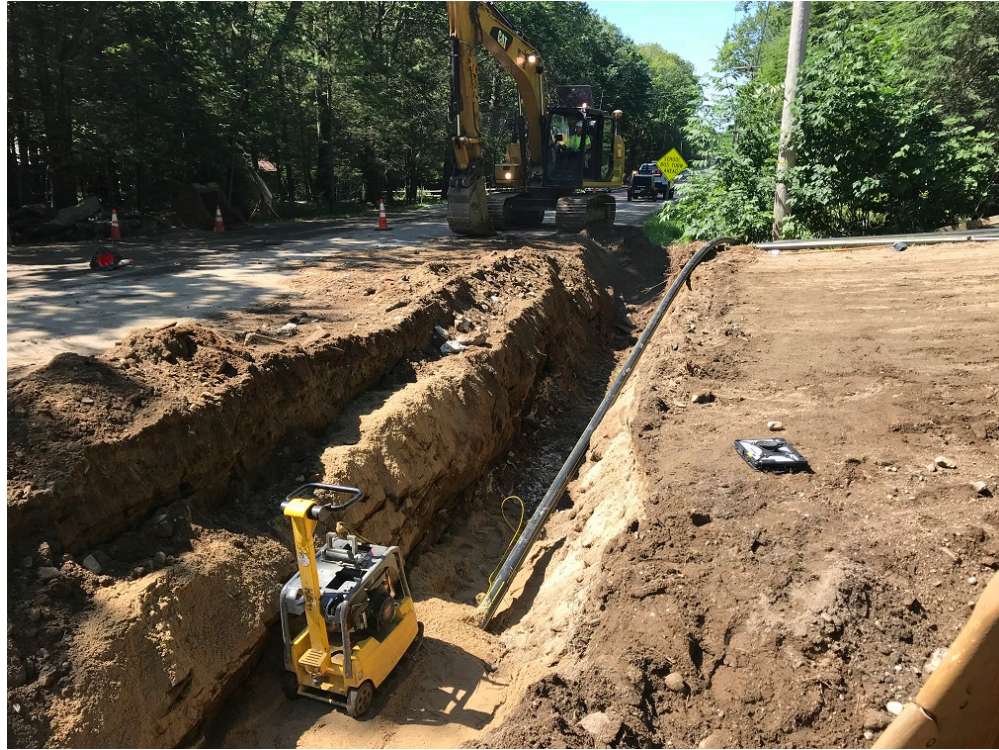
Photo 3 – Installing gas main at Falmouth Town Line
