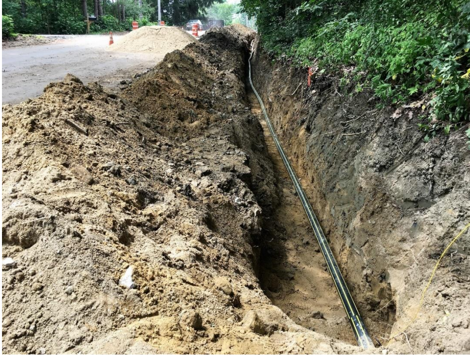
Mid-day placement of gas line from end of previous day's installation looking south prior to placement of bedding sand.
