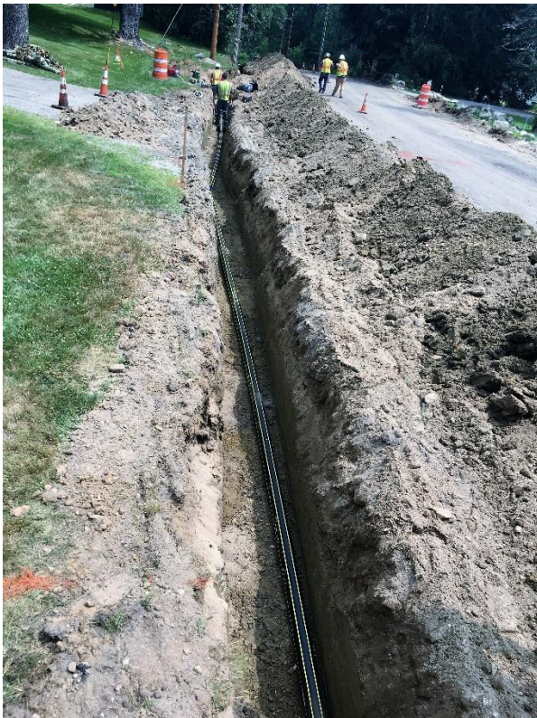
Looking north from the southern limit of progress prior to fusing pipe and backfilling.
