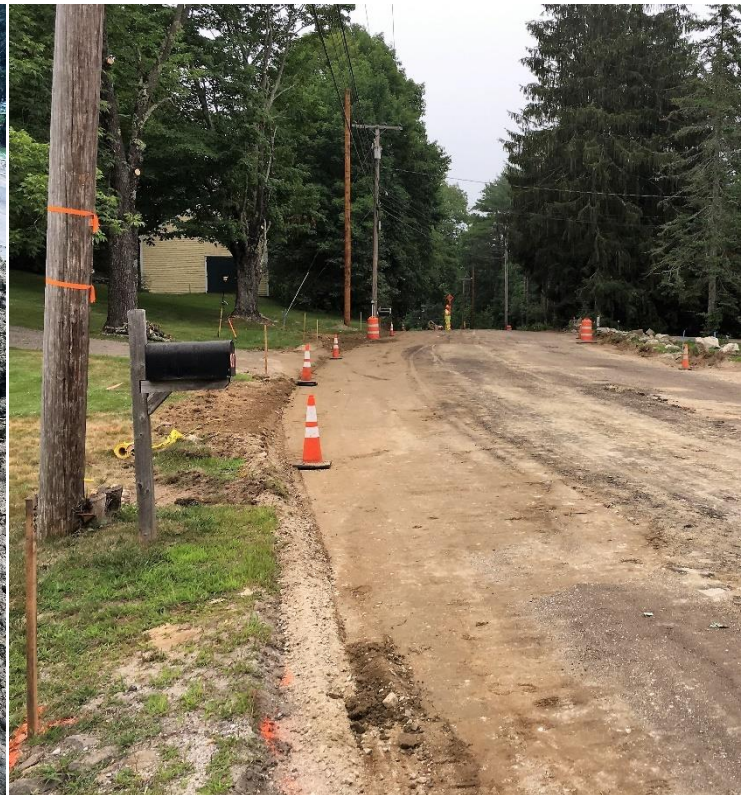
Similar view looking north of gas line backfilled to grade at the end of the day at southern end of work limits.
