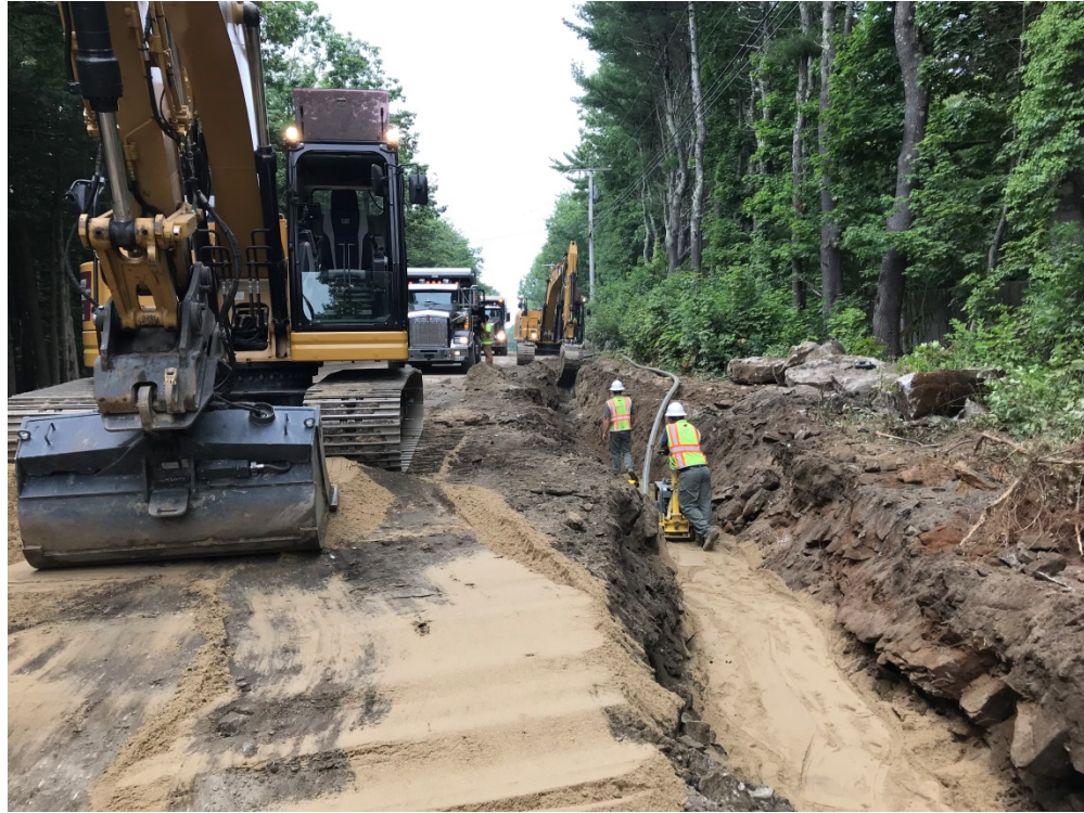
Photo 5 – Excavating for 4 inch gas main
