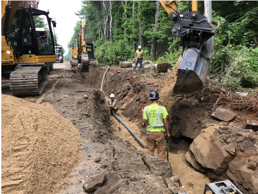
Photo 2 – Placing sand over 4 inch gas main
