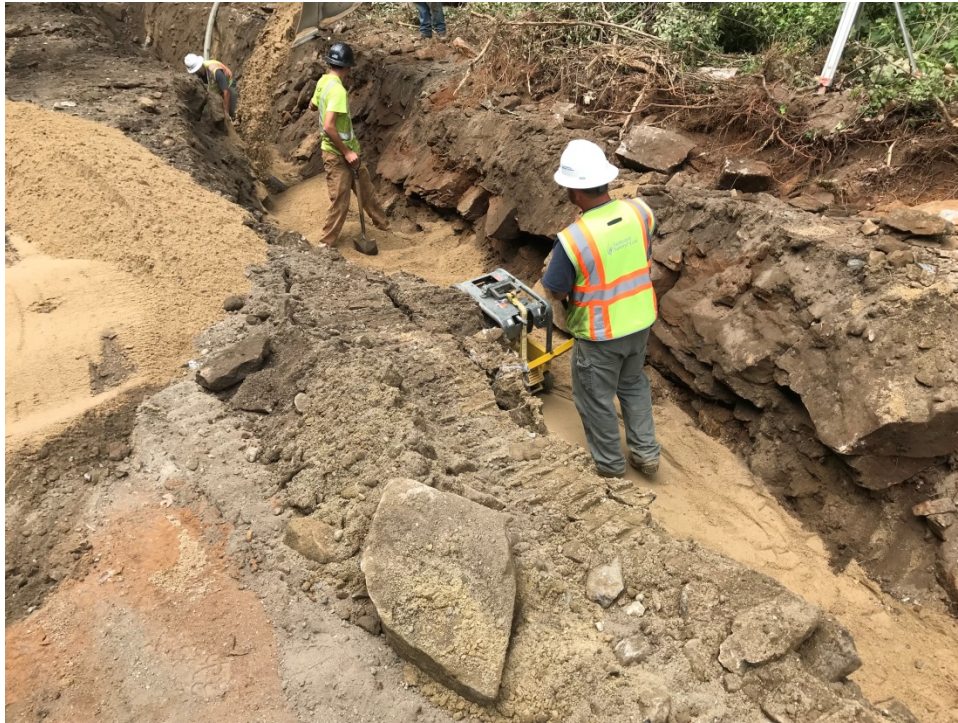
Photo 4 – Compacting sand over 4 inch gas main
