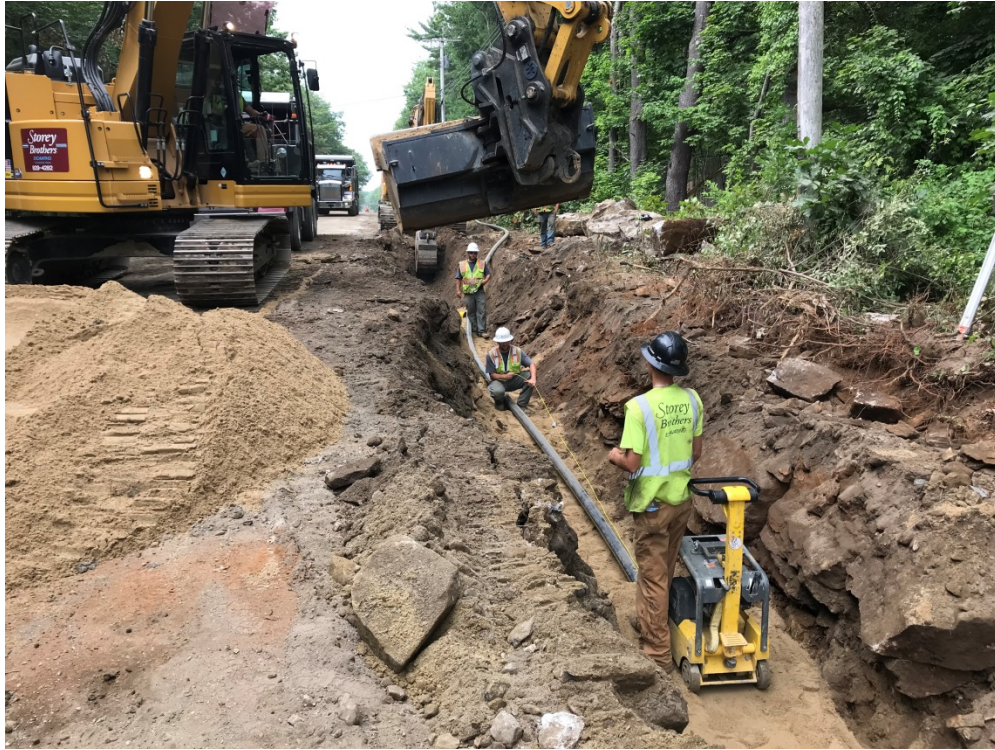
Photo 1 – Installing 4 inch gas main between 10 and 4 Middle Road
