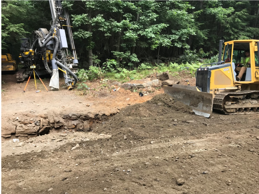
Photo 3 – Backfilling 4 inch gas main
