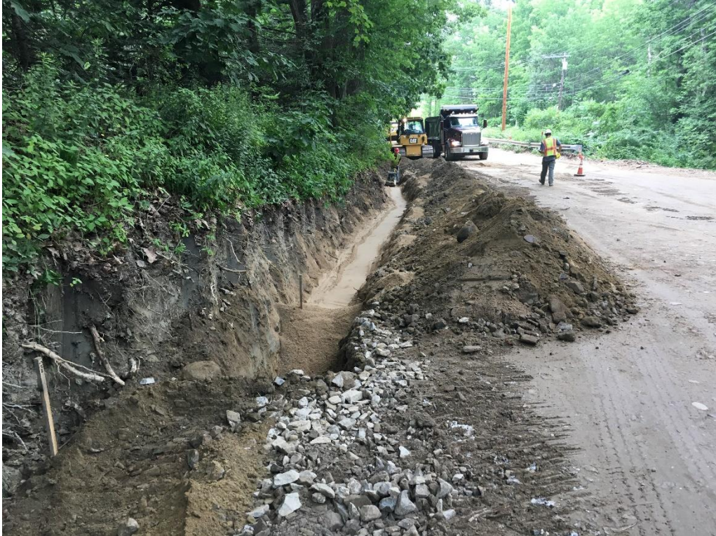
Finishing up 640 linear feet of gas main installation near the end of the day at STA 53+00.
