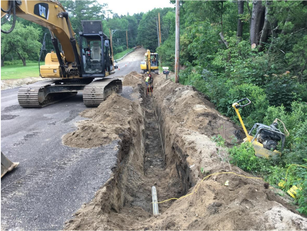
Excavating southward along western edge of road for new gas main approach gully.
