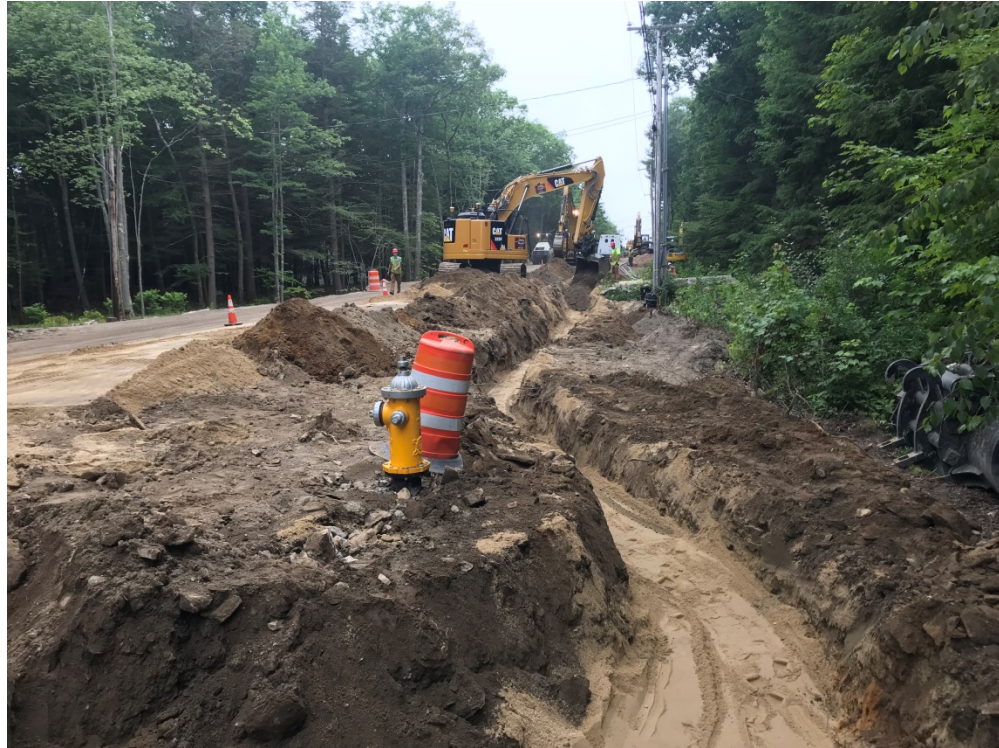
Photo 5 – Gas main trench around HYD near existing bus turnaround
