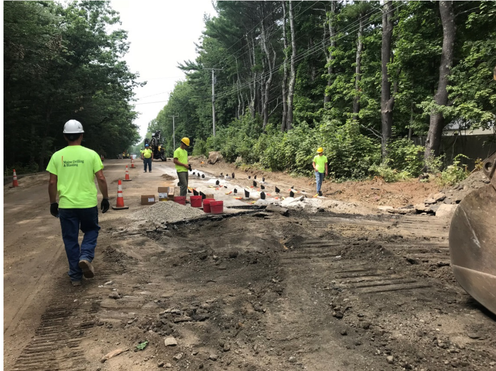
Photo 3 – Preparing to blast for gas main and underdrain near 4 Middle Road
