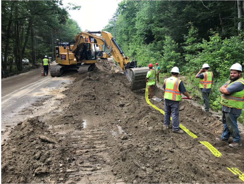
Photo 1 – Backfilling 4 inch gas main near existing bus turnaround
