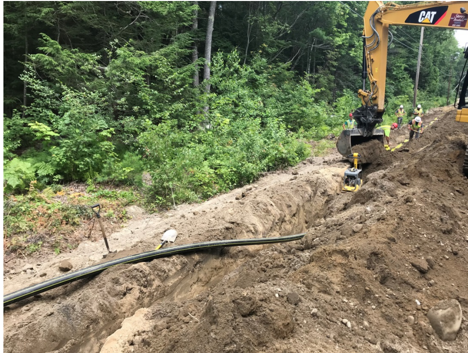
Photo 4 – Backfilling gas main near 10 Middle Road
