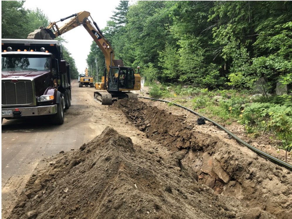
Photo 2 – Excavating for 4 inch gas main
