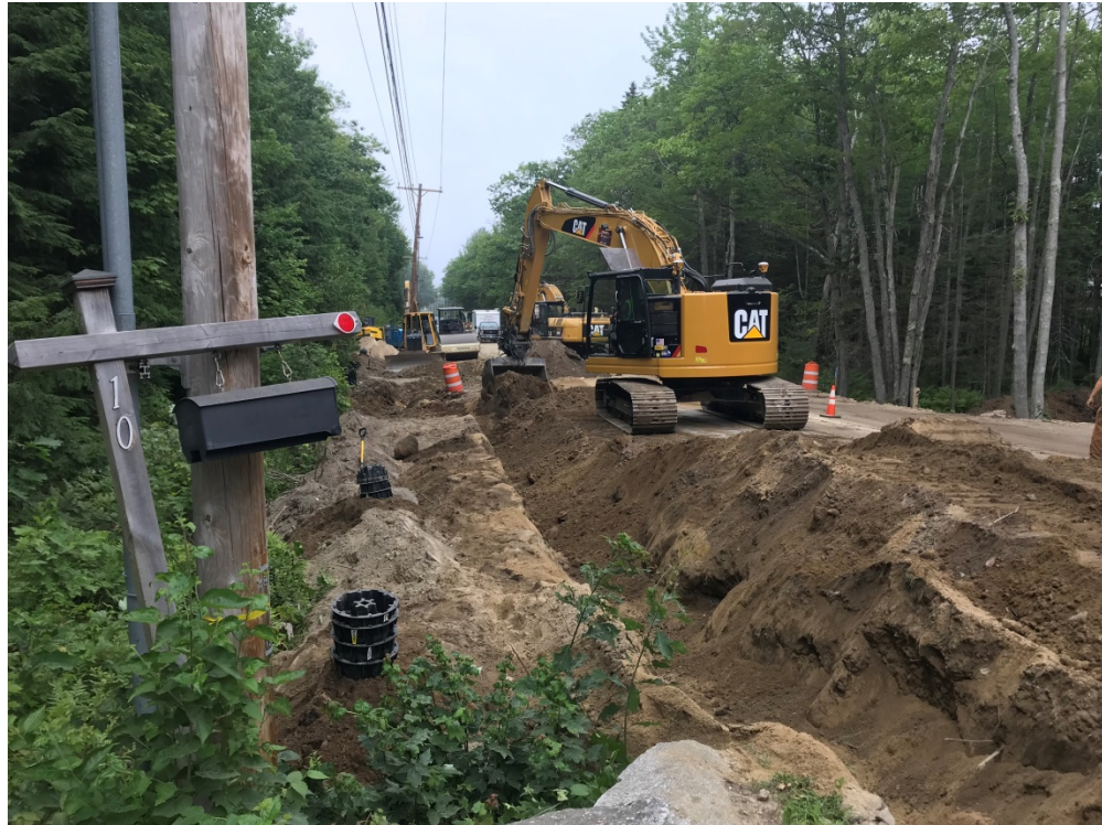
Photo 6 – Backfilling 4 inch gas main near existing bus turnaround
