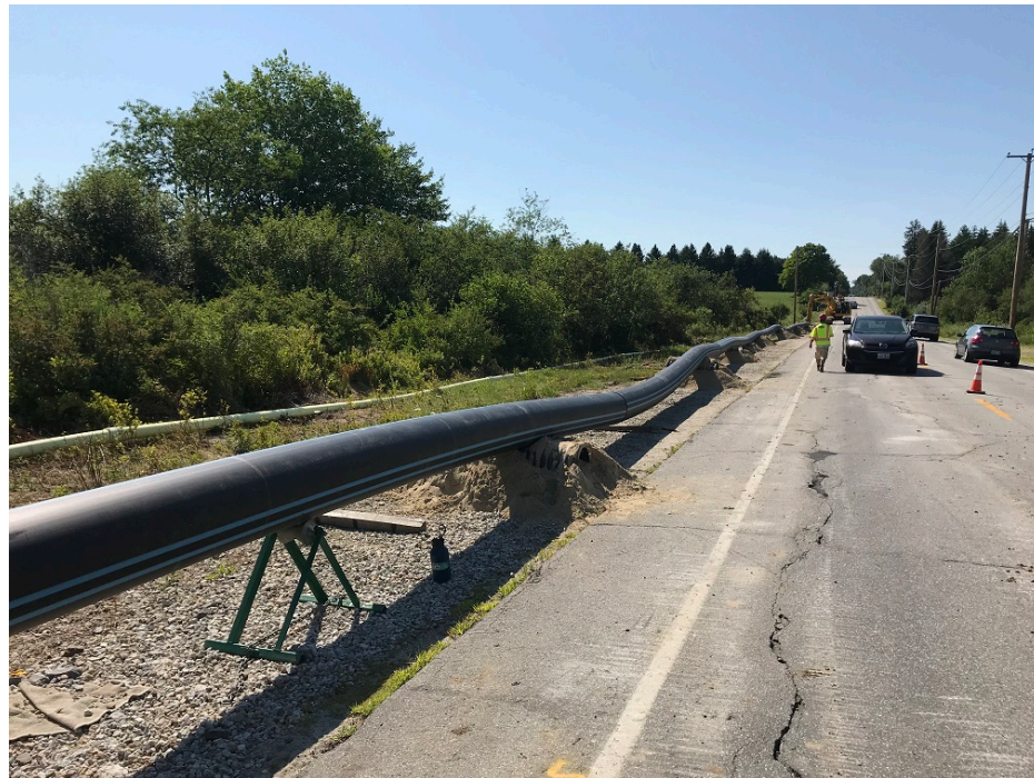
Photo 2 – Fused 16 inch HDPE water main
