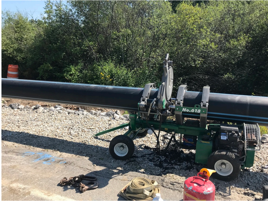
Photo 1 – 16 inch HDPE water main in fusing machine
