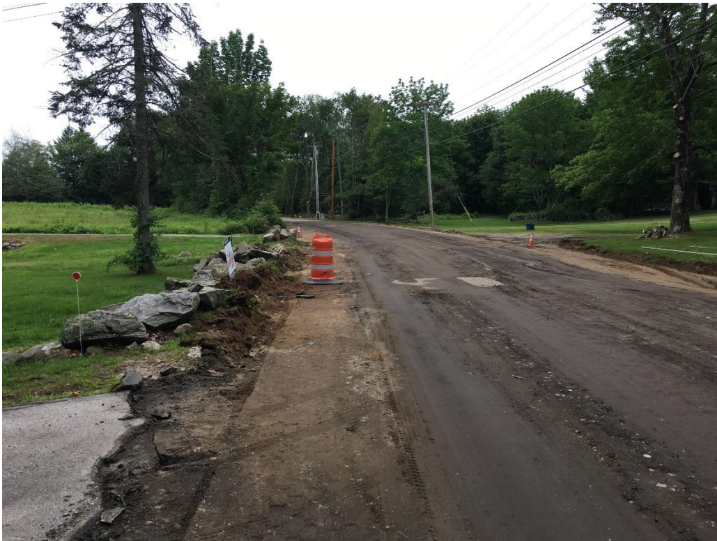
Finished pavement removal and grubbing on the eastern side of road by the end of the day.
