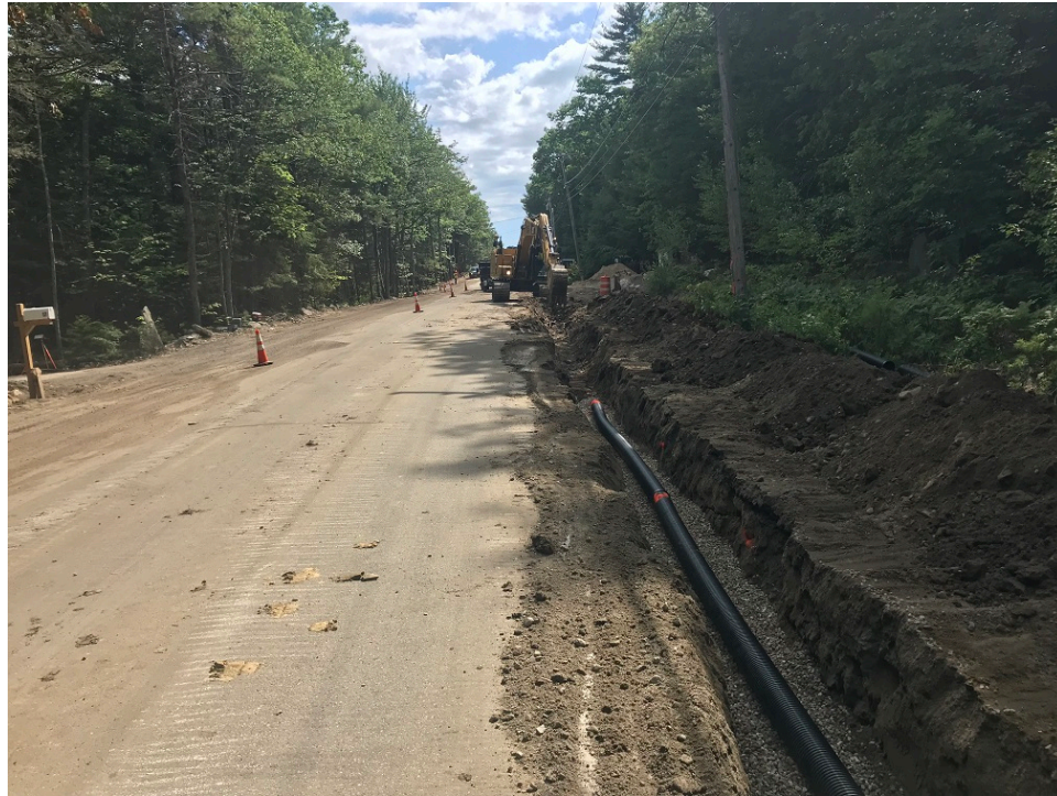
Photo 4 – Excavating for 4 inch underdrain near existing bus turnaround
