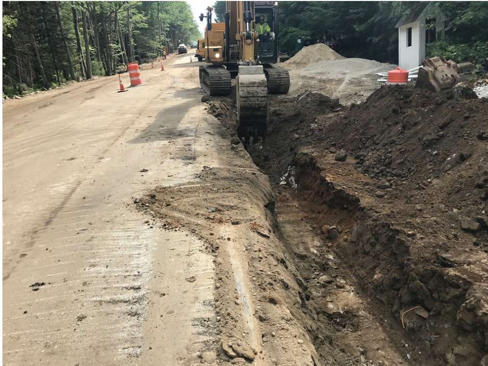
Photo 6 – Excavating for 4 inch underdrain near existing bus turnaround
