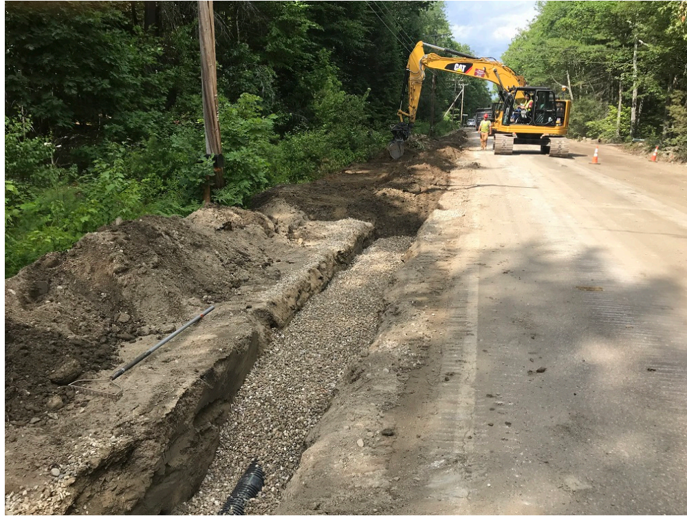
Photo 3 – Backfilling 4 inch underdrain near 23 Middle Road
