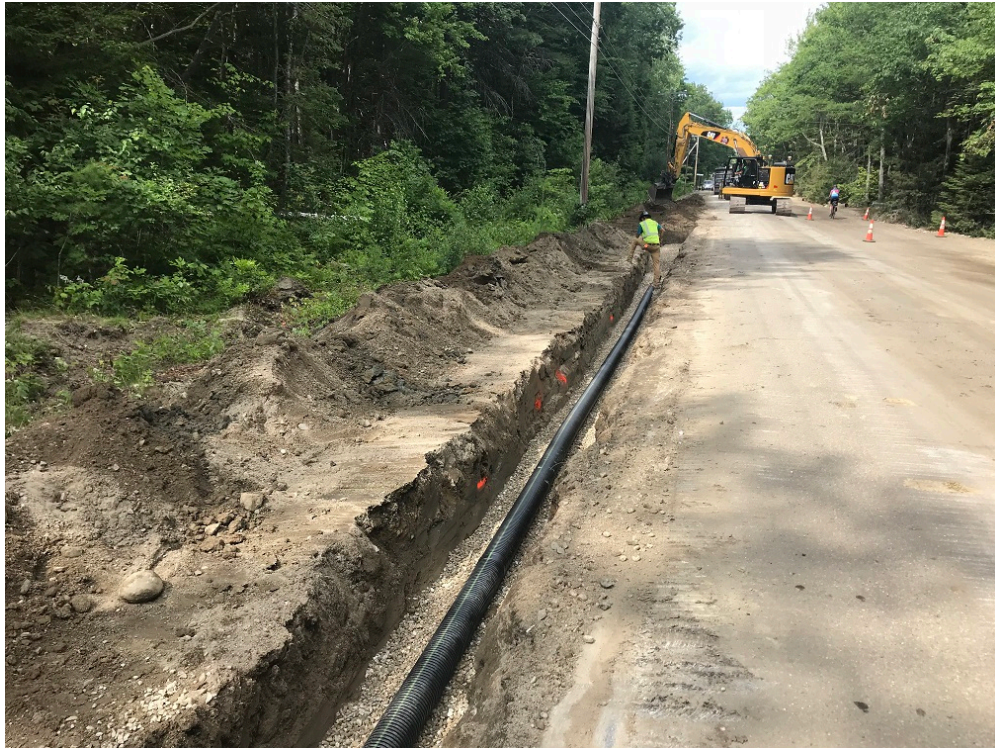
Photo 2 – Installing 4 inch underdrain near 23 Middle Road
