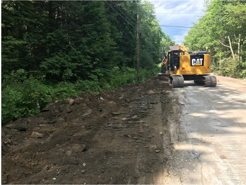
Photo 5 – Cleaning up edge of road after underdrain installation
