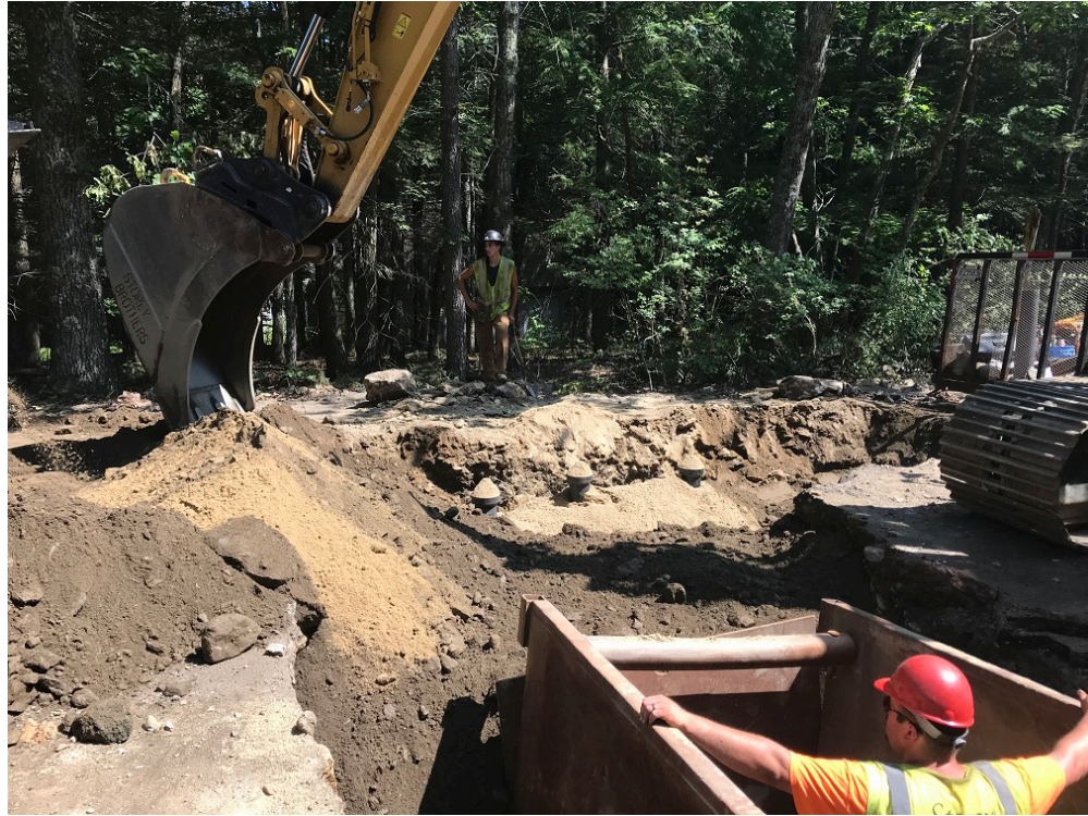
Photo 5 – Backing filling around valve boxes for HYD at STA 0+85
