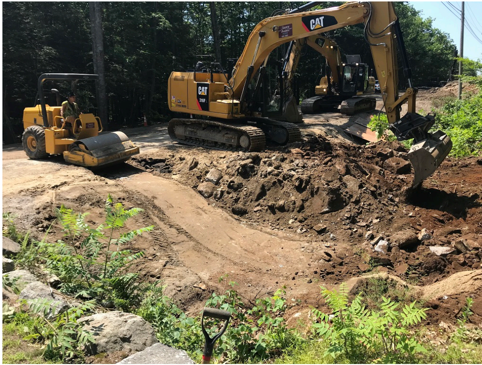
Photo 1 – Backfilling and compacting water service trench at 10 Middle Road
