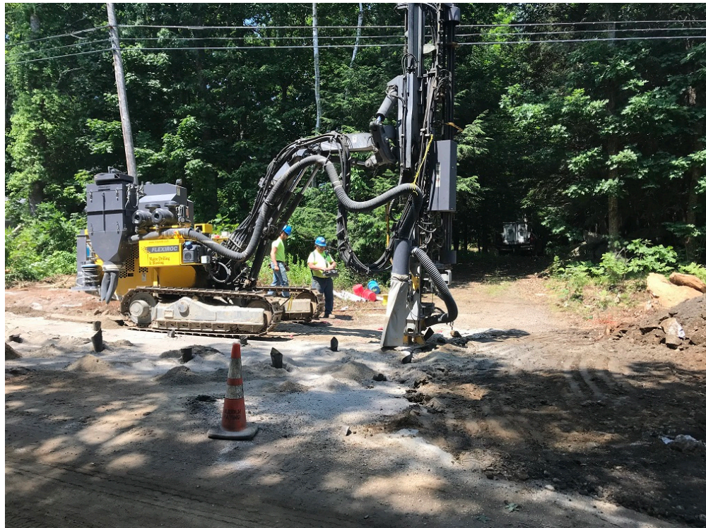
Photo 6 – Drilling for bedrock between 10 Middle Road and 4 Middle Road
