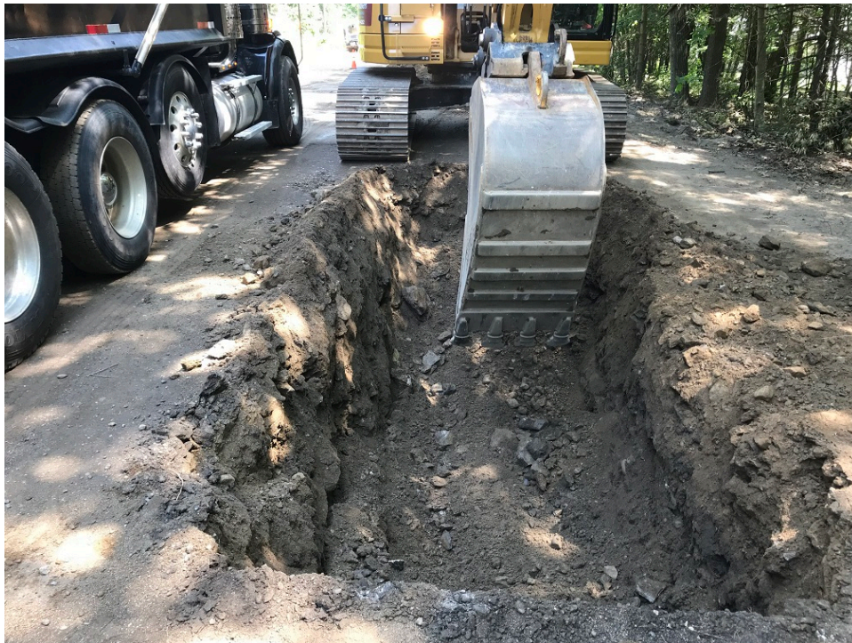
Photo 4 – Excavating for HYD installation at STA 0+85
