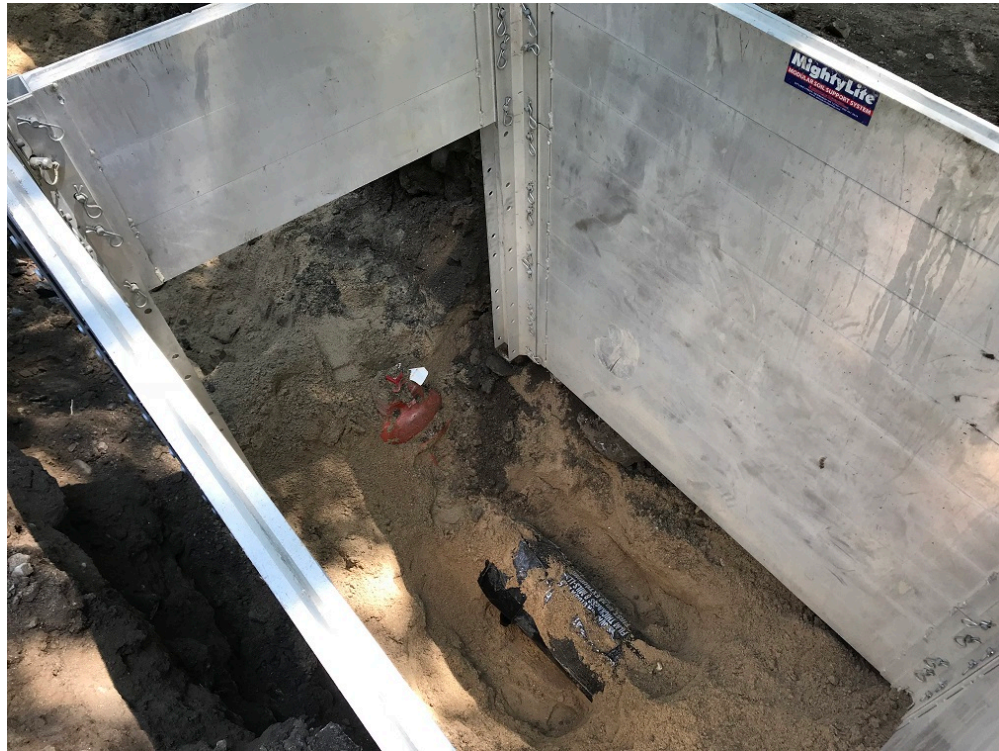
Photo 5 – 12 inch gate valve and pipe exposed at STA 0+85 for HYD installation
