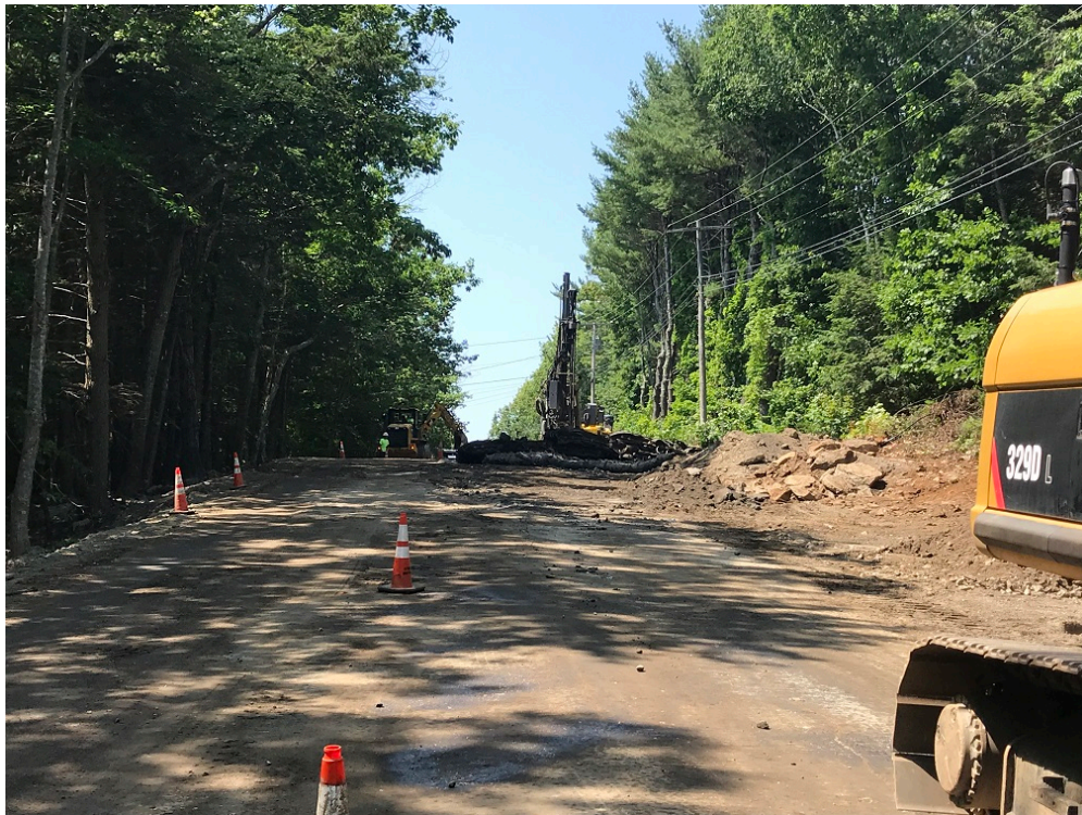
Photo 2 – Preparing for blast in front of 10 Middle Road
