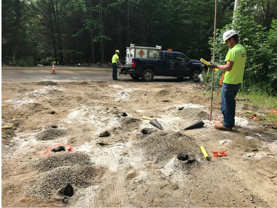
Photo 1 – Loading for blast at bus turnaround at 4 Middle Road
