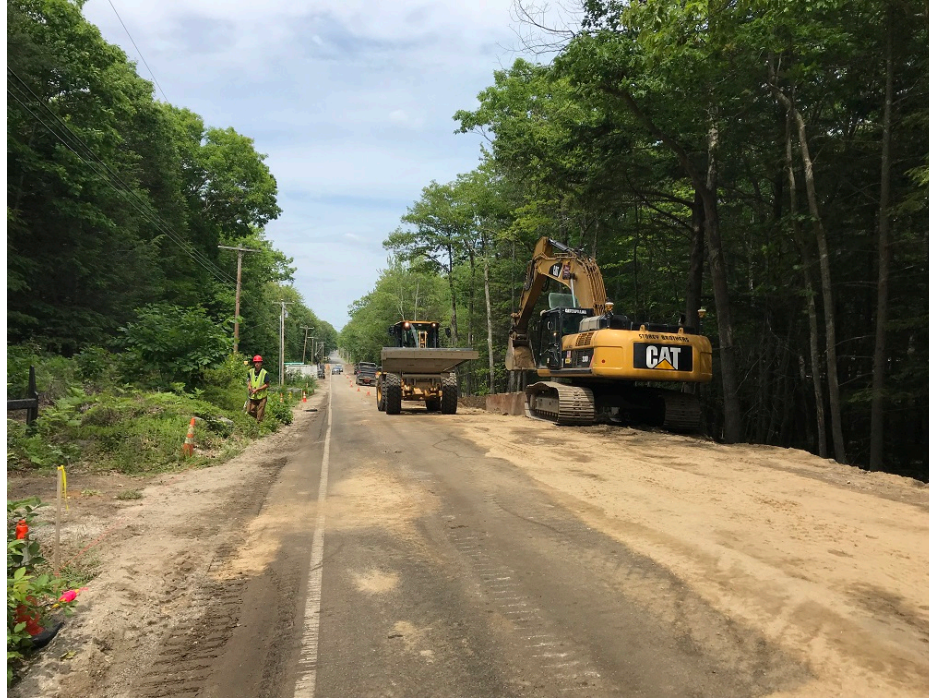
Photo 5 – Placing sand for 12 inch water main
