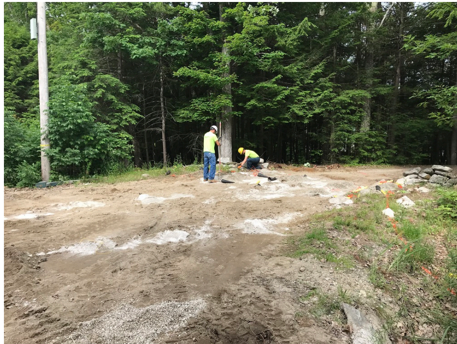
Photo 2 – Loading for blast at bus turnaround at 4 Middle Road
