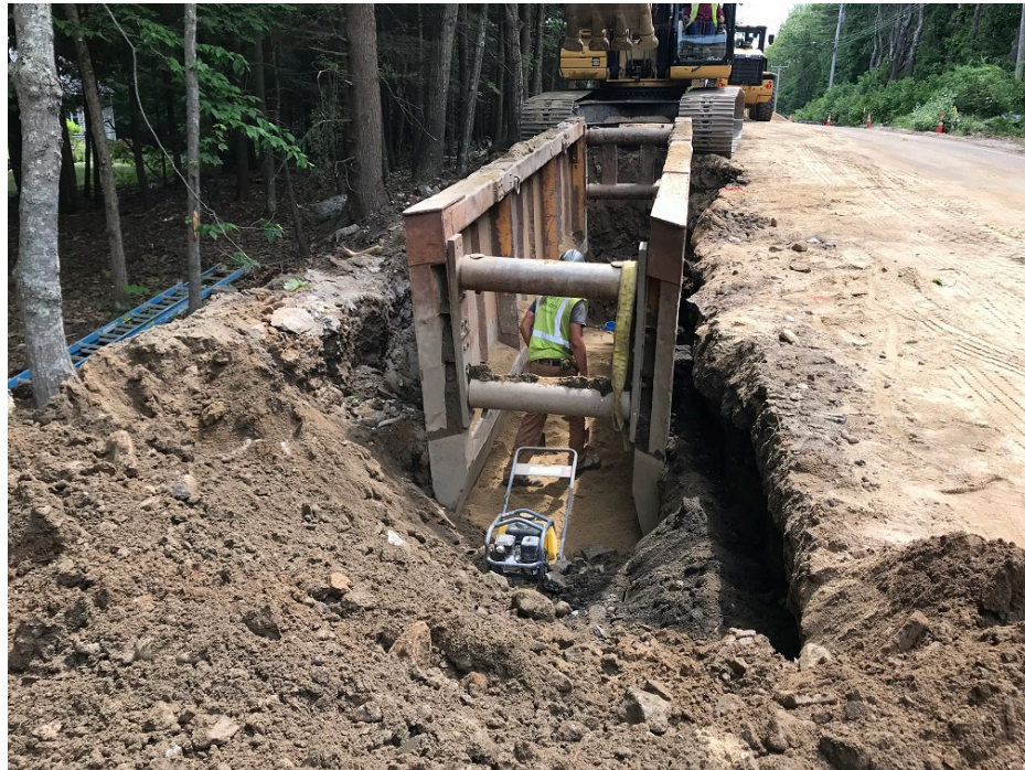
Photo 6 – Installing 12 inch water main
