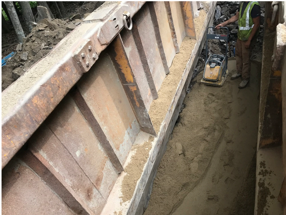
Photo 8 – Compacting sand bedding for 12 inch water main near Tall Pines Way
