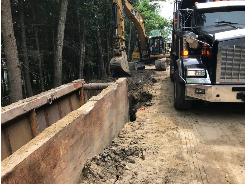
Photo 7 – Excavating for 12 inch water main near Tall Pines Way
