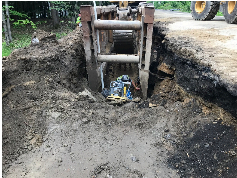
Photo 3 – Placing sand bedding for 12 inch water main near 15 Middle Road
