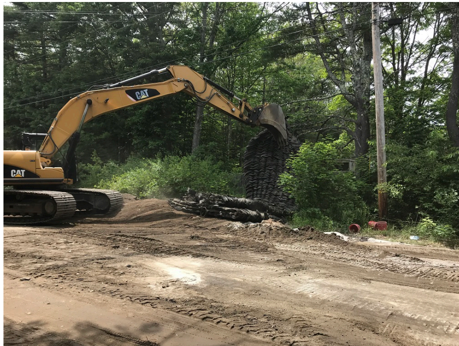
Photo 4 – Placing blasting mats for water service at 4 Middle Road
