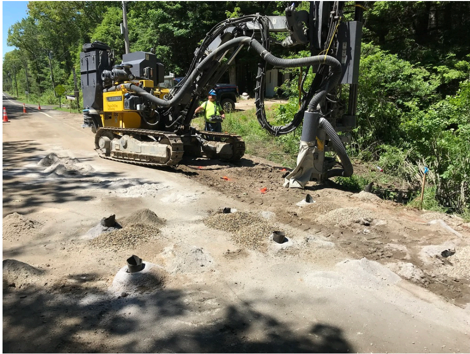
Photo 1 – Drilling bedrock for gas main on west side of the road near 4 Middle Road
