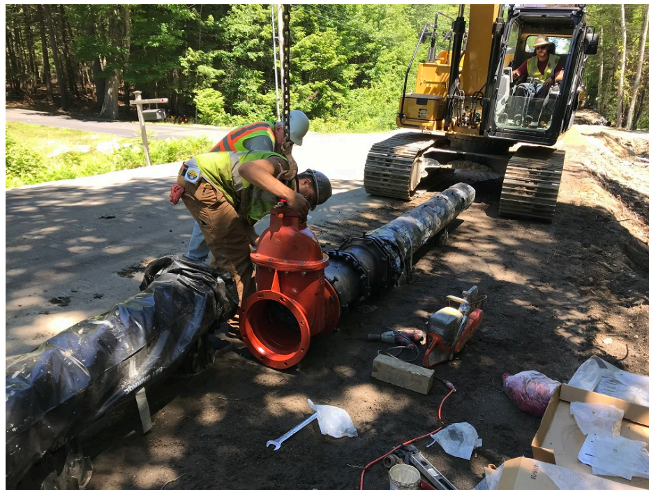
Photo 2 – Assembling 12 inch gate valve and 6 X12 tee with 6 inch gate valve for hyd
