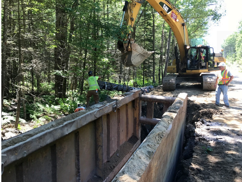
Photo 5 – Installing 12 inch water main
