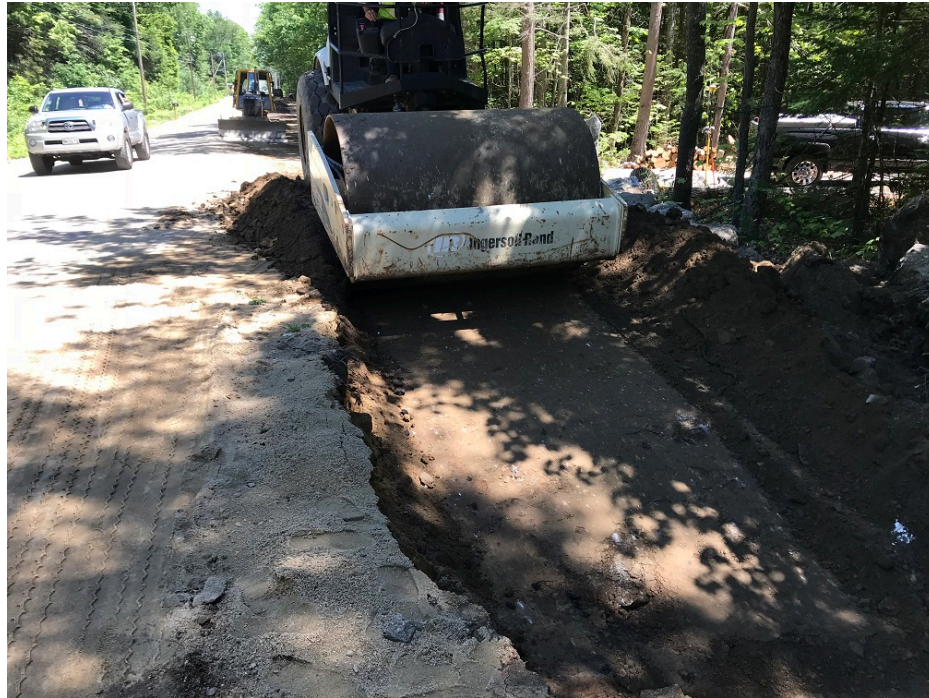
Photo 3 – Backfilling and compacting water main trench
