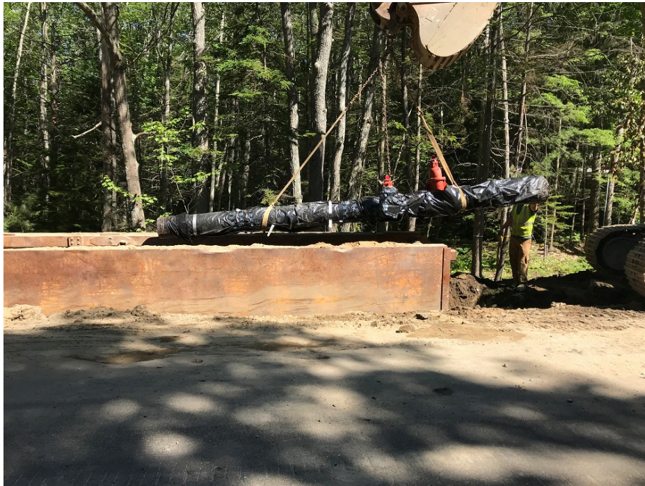
Photo 8 – Installing 12 inch water main with valve assembly near 15 Middle Road
