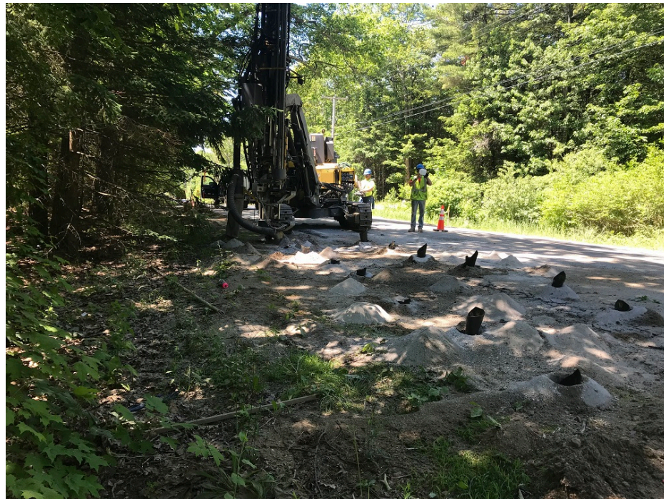
Photo 2 – Drilling for second blast of the day just south of Tall Pines Way
