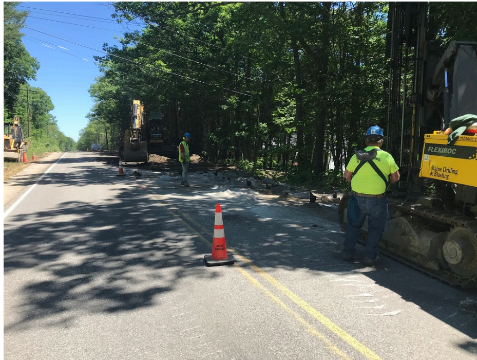
Photo 3 – Drilling for second blast of the day just south of Tall Pines Way
